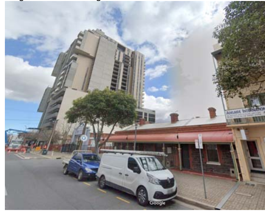
Wright Street – looking West towards Whitmore Square
