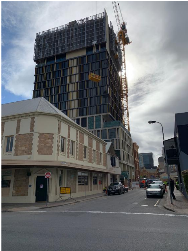
Image 7 - Currently under construction the 16 storey Indigo Hotel in Market Street.
