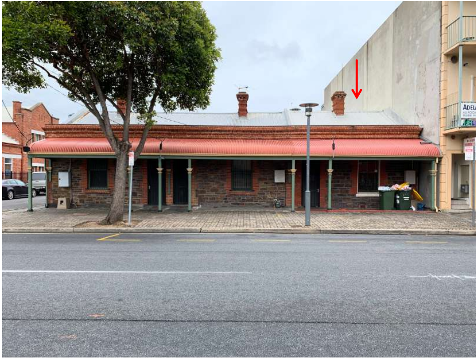
Figure 7: 134, 136, 136a Wright Street. 134 to right hand side.
