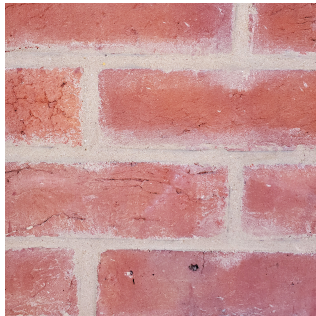
EXISTING RED BRICK LOCATION: WINDOW & CORNER QUINS
