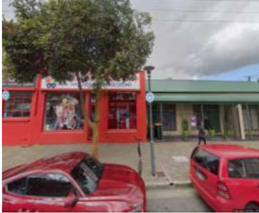
Wright Street - looking South
