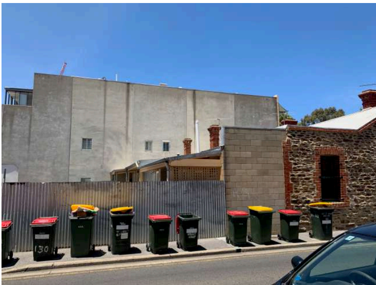
Neighbouring eastern boundary wall
