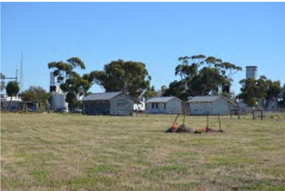
Figure 4.4 : Overview of the three animal quarantine buildings (Structures 1, 2 and 3), facing north east.
