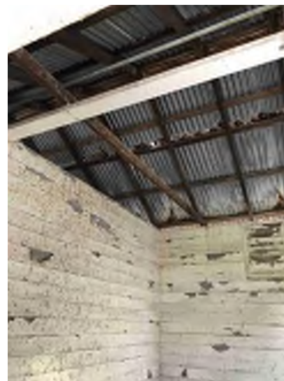
Figure 3.17: Corrosion of Roof Sheetting
