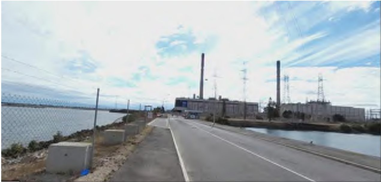
Plate 5-3 QPS Main Access Gate
