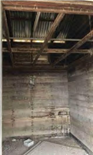
Figure 3.12: Staining on Internal Timber Planks
