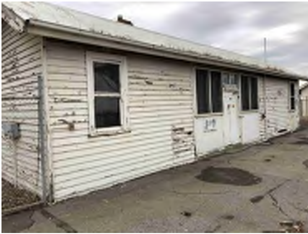
Figure 3.5: General Photo of Weatherboard Condition
