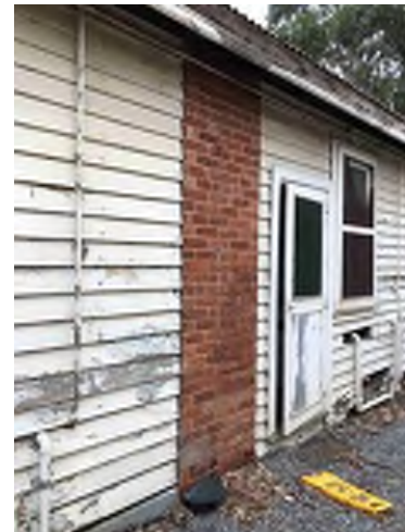
Figure 3.2: Brick Chimney in Building 1
