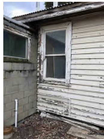
Figure 3.4: Example of Deteriorated Weatherboard
