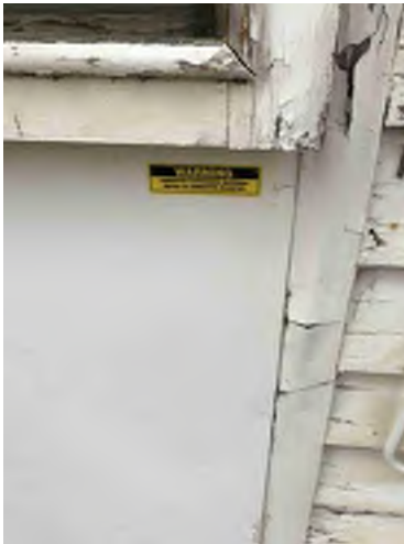
Figure 3.7: Asbestos Warning Labels
