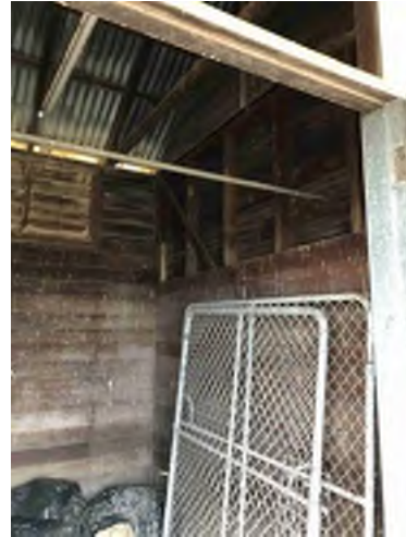
Figure 3.9: Timber Frame of Building 2
