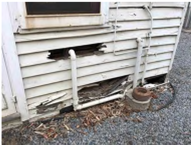
Figure 3.3: Exposed Timber Frame and Missing Cladding
