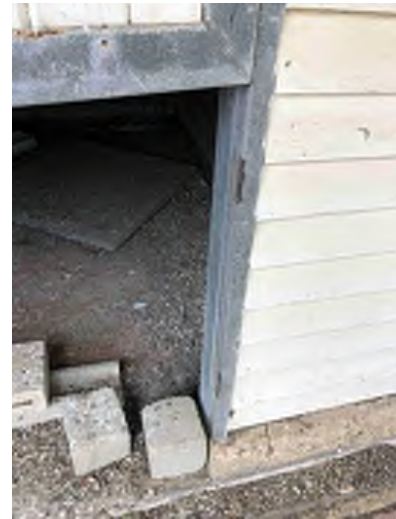
Figure 3.13: Damaged/Missing Doorway Brackets
