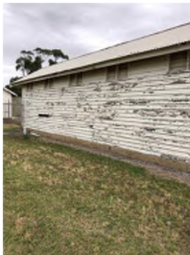
Figure 3.10: Weatherboard Cladding of Building 2
