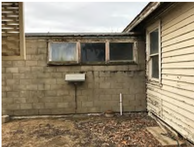
Figure 3.1: Blockwork Structure Attached to Building 1
