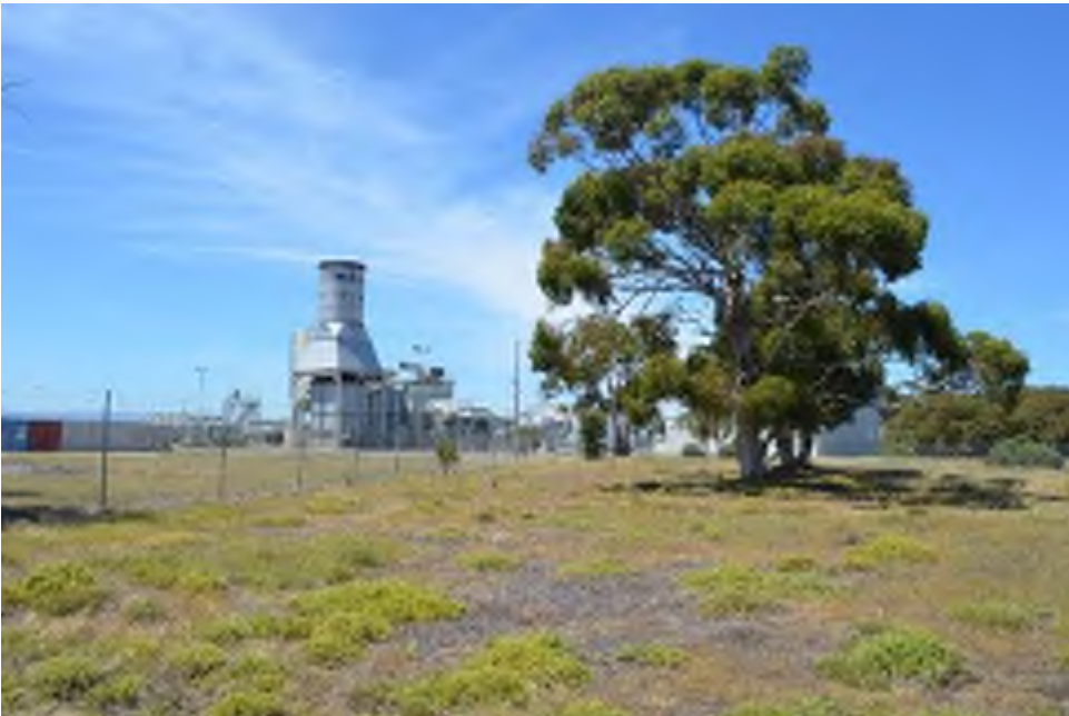
Figure 4.3 : View of proposed laydown area within the Quarantine Station State Heritage Place boundary, facing south.
