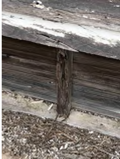
Figure 3.14: Deterioration of Timber Frame
