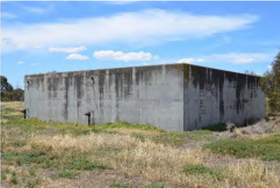
Figure 4.10 : Reinforced concrete water tank (Structure 5), facing northeast.
