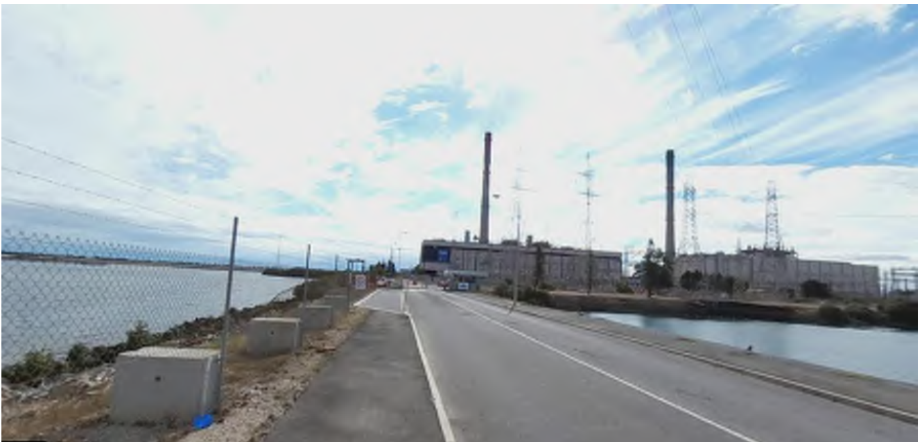
Figure 2-1: Main access gate
