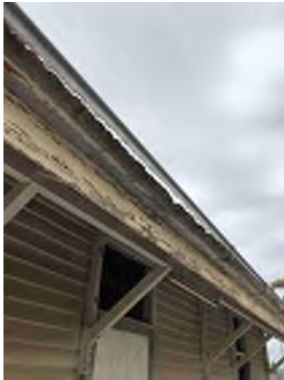
Figure 3.18: Holes Forming in Gutters from Corrosion
