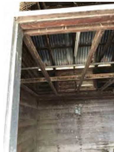
Figure 3.11: Internal View of Roofing
