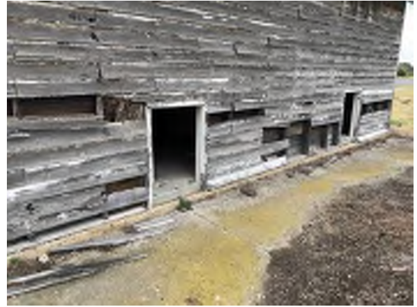
Figure 3.15: Severe Degradation of Weatherboard Cladding
