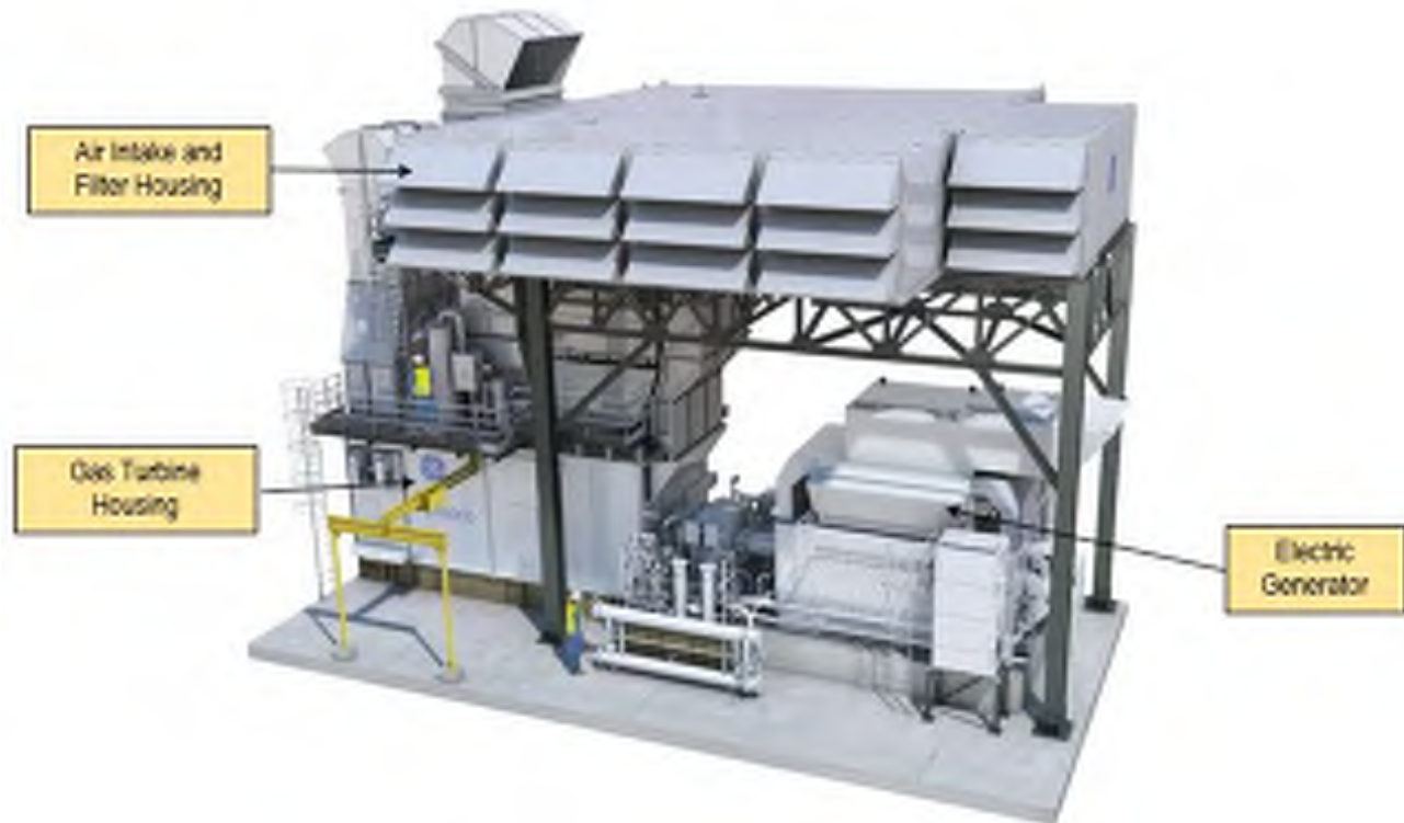
Figure 4-4 Gas turbine and generator package layout
