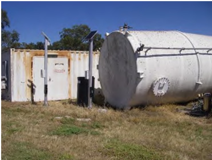
Plate 5-6 Disused demineralised water storage tank and hazardous materials shipping container
