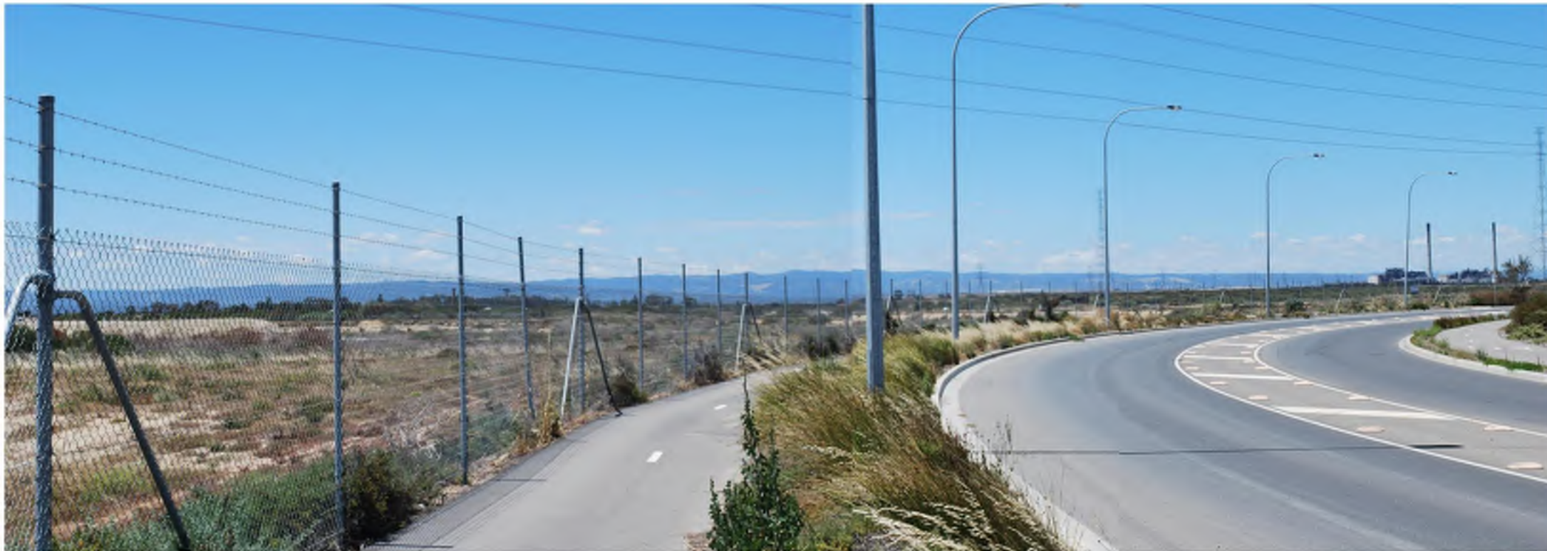
Photo: Mersey Road. View south east to existing Quarantine Power Station.
