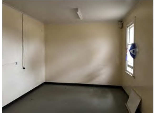
Figure 3.6: Building 1 Internal Fit Out
