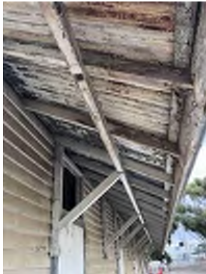
Figure 3.16: Deterioration of Roofing Frame
