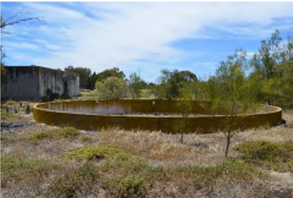
Figure 4.9 : Reinforced concrete circular water tank (Structure 4), facing north.
