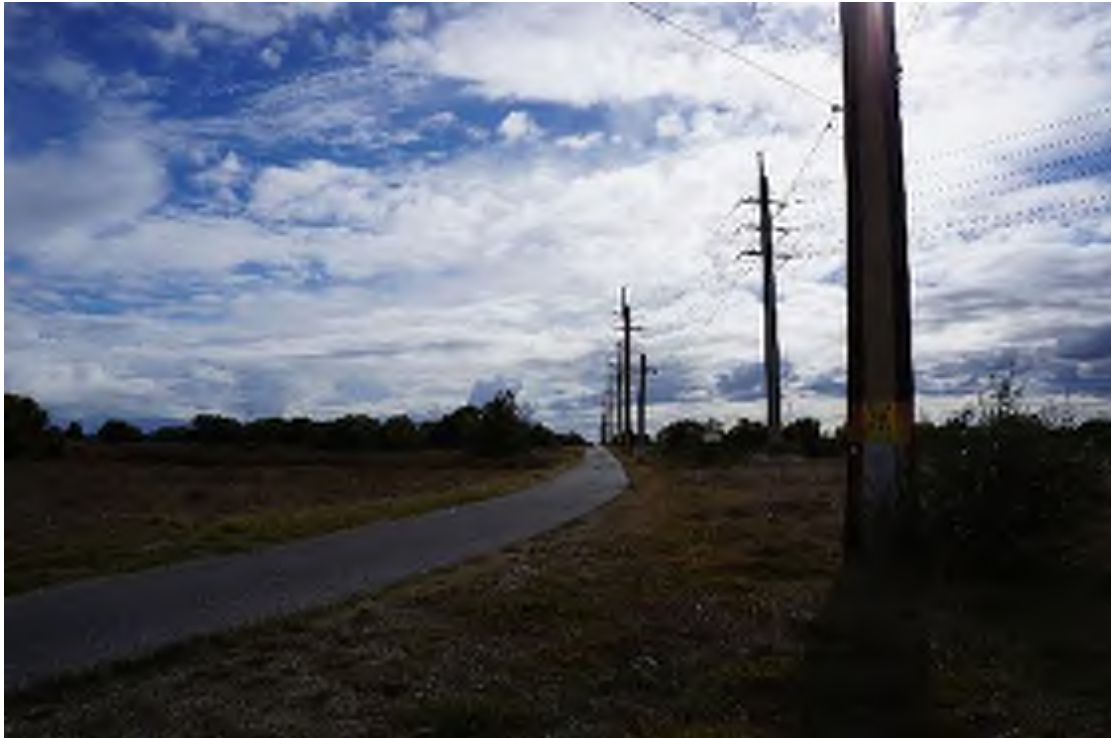
Plate 3-3 access road to QPS with adjacent 66kV transmission, looking north
