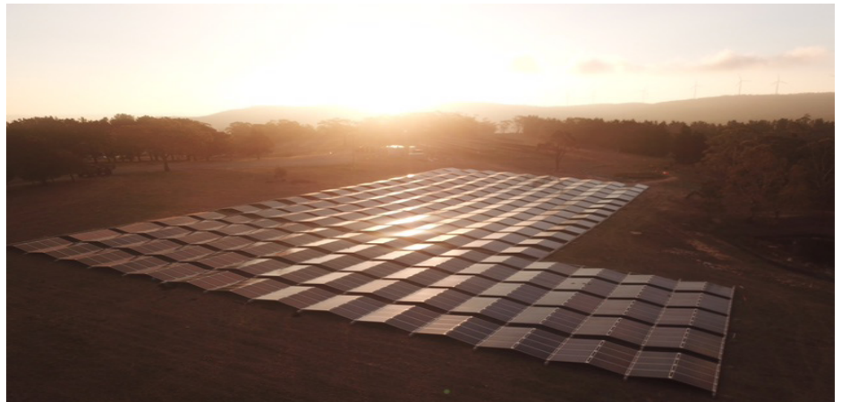
Example of a LMS Landfill Solar System
