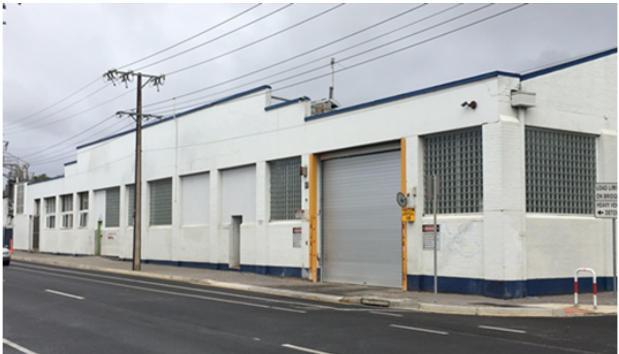
Leader Street Façade
