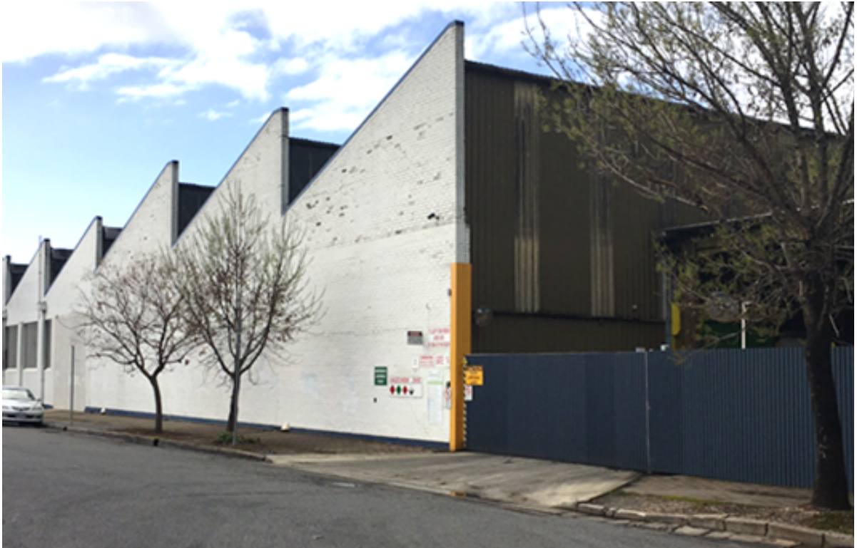
First Avenue Façade
