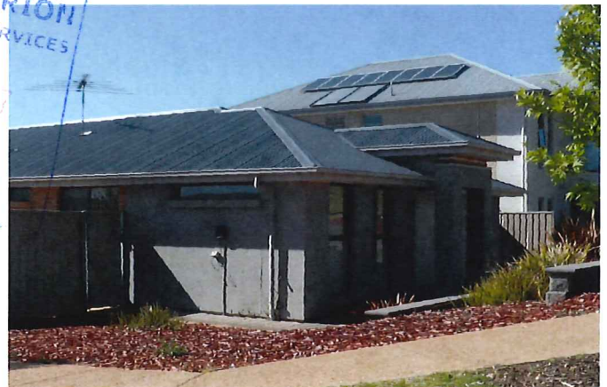
X High level windows on large blank walls are not acceptable.
