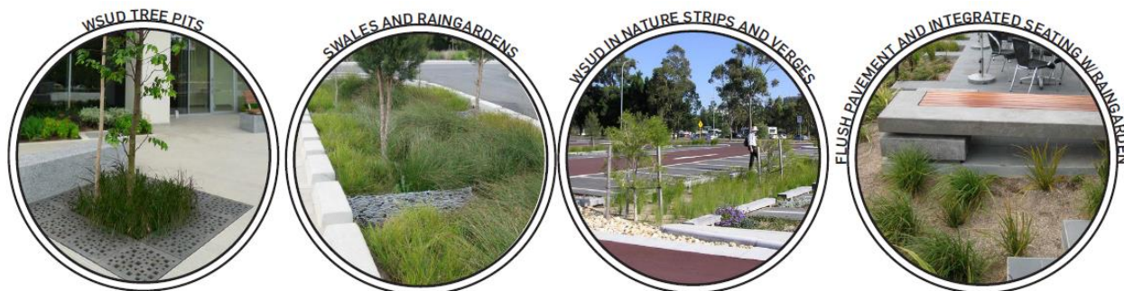
Figure 11 – Examples of proposed kerb inlet swales and raingardens
