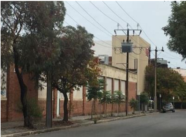
Picture 4 – Existing site, viewed west from Maple Avenue
