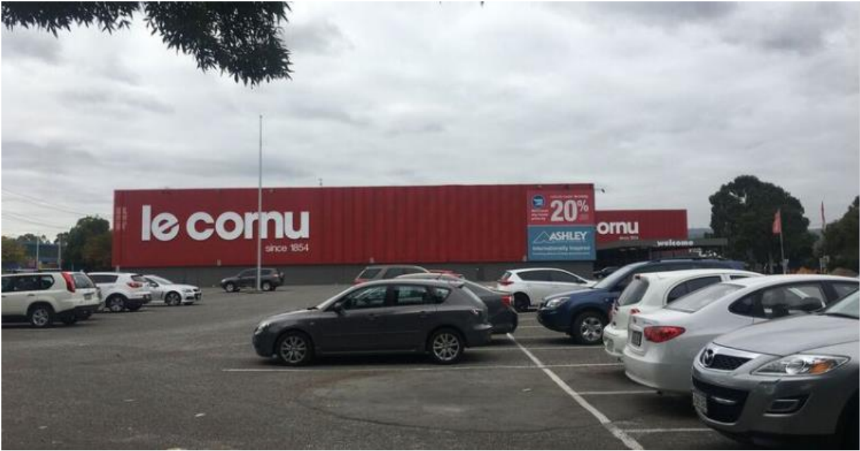
Picture 1 – Subject site, existing conditions viewed east from Anzac Highway
