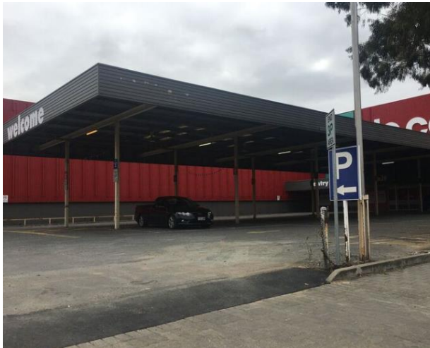
Picture 3 – Existing undercover car parking on site
