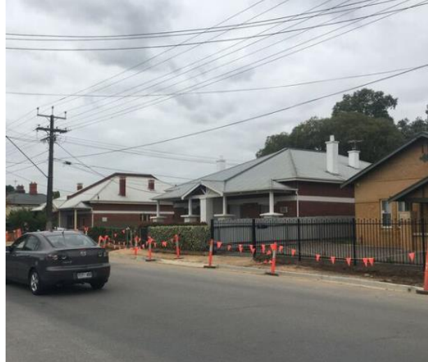
Picture 11 – Single storey dwellings on the southern side of Leader Street
