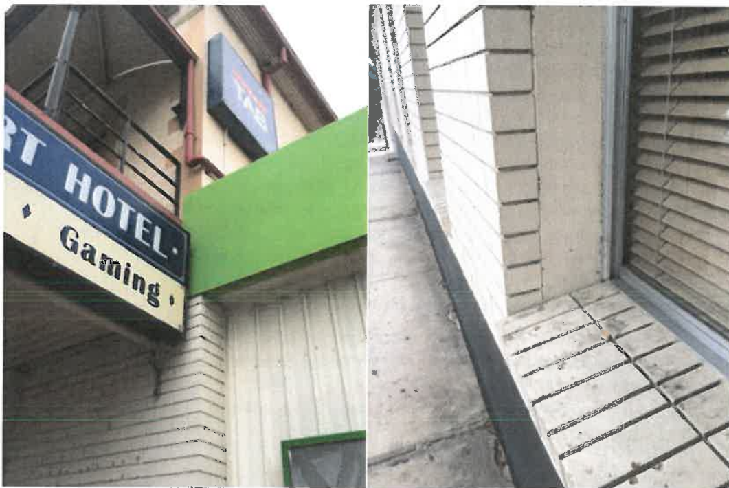
Figure 15 (Left) Detailed View showing build out of Ground Floor brick skin Source: Flightpath Architects 28 September 2016
