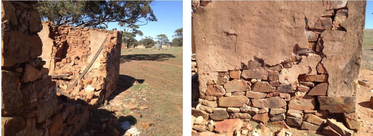
Figure 6 Photographs of Tarcowie siltstone used in building construction
