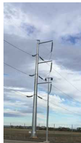
TYPICAL PHOTO - SINGLE CIRCUIT POLE
