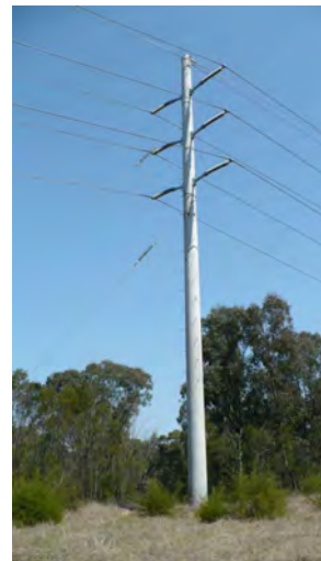
TYPICAL PHOTO - DOUBLE CIRCUIT POLE
