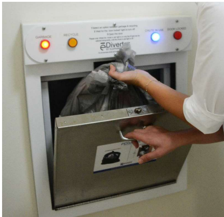
Figure 5-6: Example of e-diverter disposal access point in Residential local disposal rooms for waste / recycling disposal on residential levels. Source: http://www.elephantsfoot.com.au/products/chutes/waste-and-recycling-diverter
