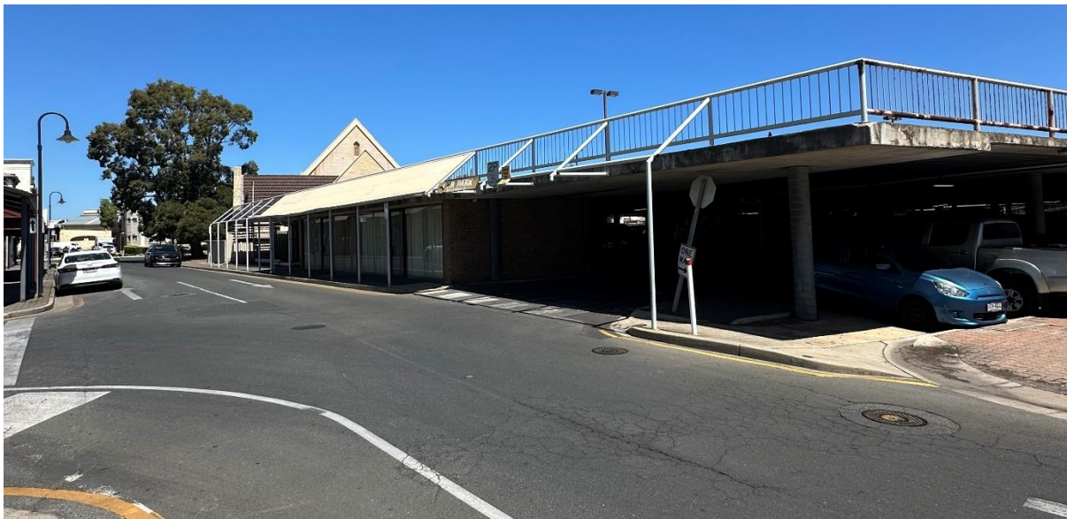
Figure 5.2 View from Marryatt Street that shows the two-level car park structure to be removed
