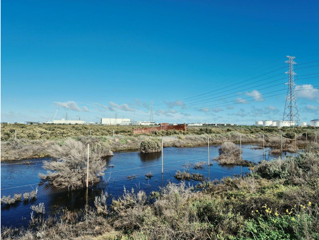
Figure 5: seawater ponding after overtopping northern bank 18.6.2026
