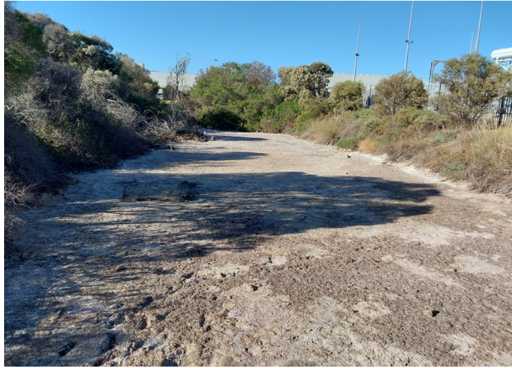
Figure 4 - Existing retention pond
