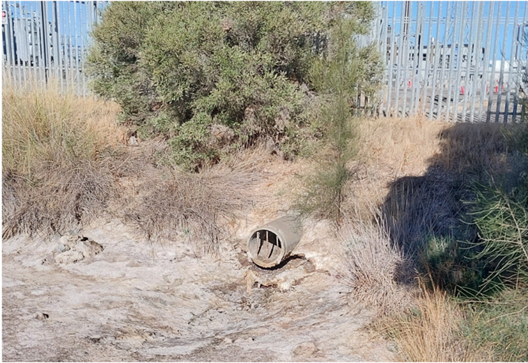
Figure 8 - Existing retention pond 450mm RCP stormwater inlet pipe
