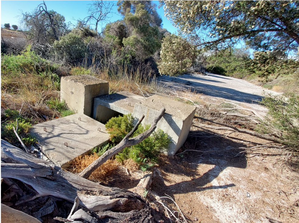
Figure 6 - Figure 5 - Existing retention pond overflow RCBC (2)
