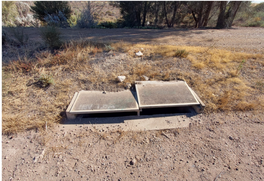
Figure 9 - Existing SEP - northern side of existing access track
