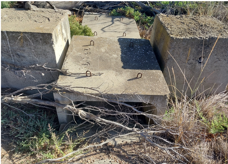
Figure 5 - Existing retention pond overflow RCBC (1)
