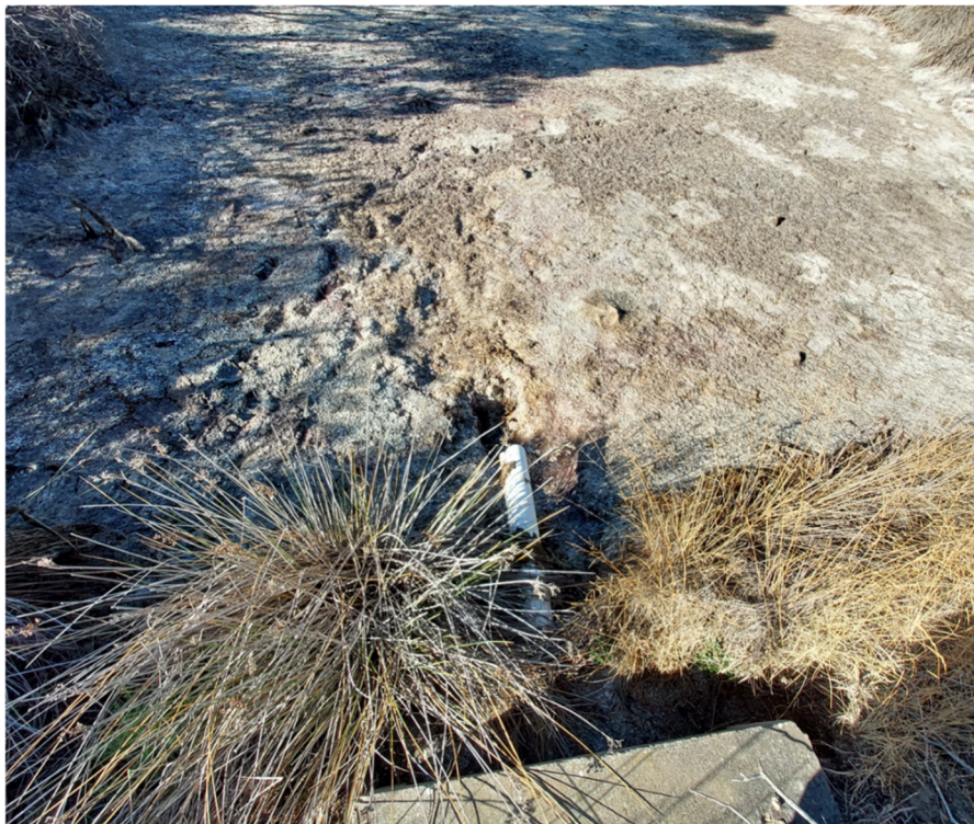
Figure 7 - Existing PVC pipe at retention pond overflow RCBC location
