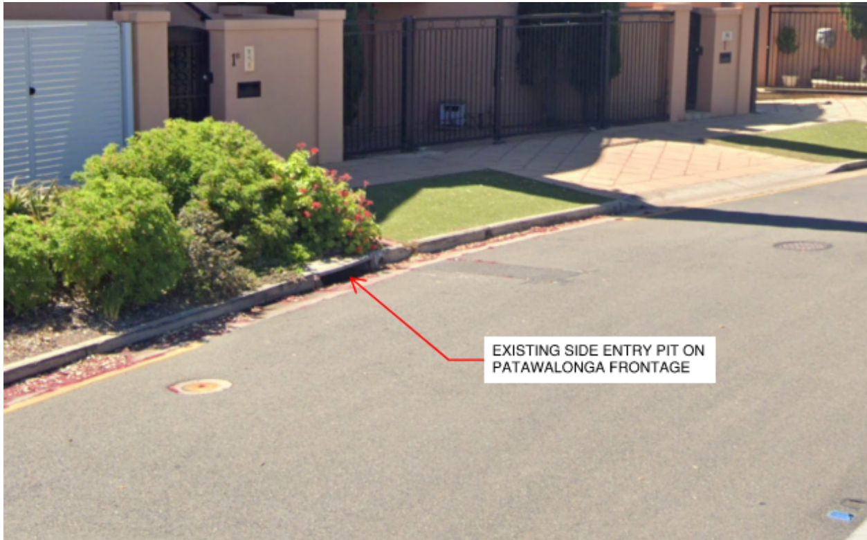
Figure 2 Existing Council Side Entry Pit
