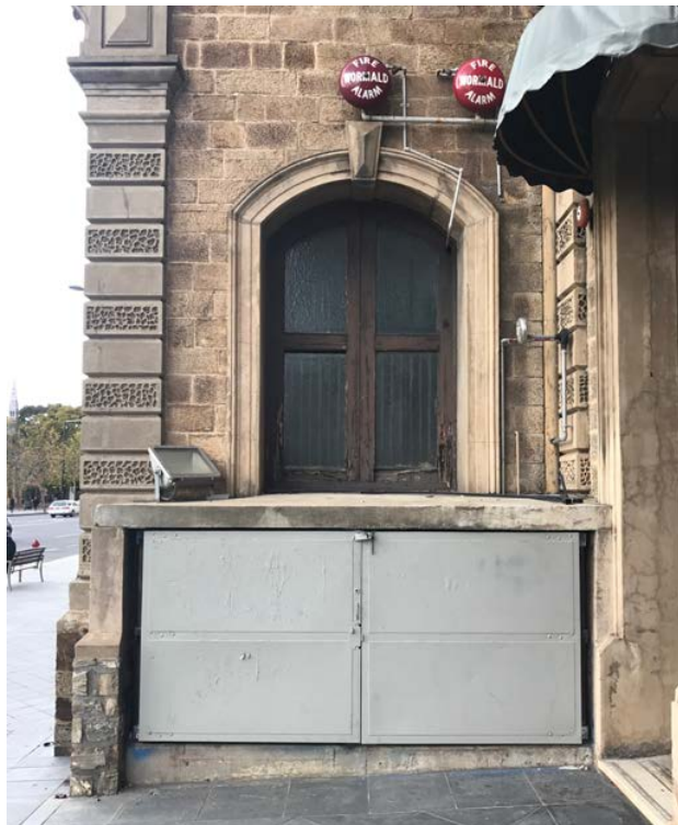
IMAGE 08 – Fire Booster Box abutting the subject site but located within the adjoining property.
