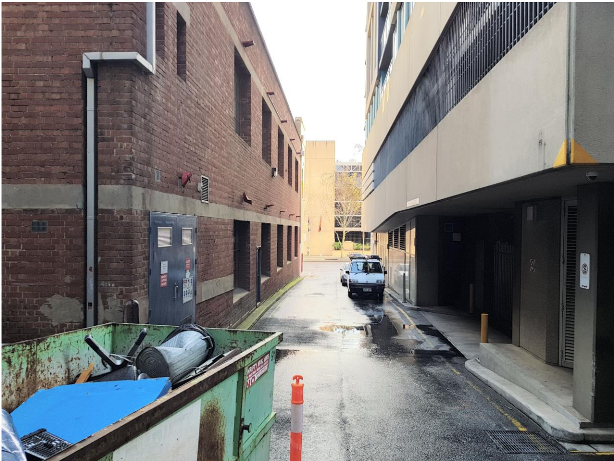
Bernath Place – view to North Terrace from south
