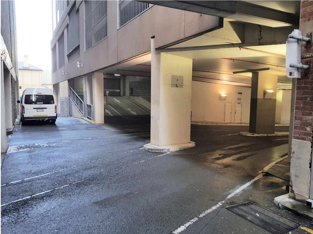
Continuation of Bernath Place across car park driveway – view to northwest
