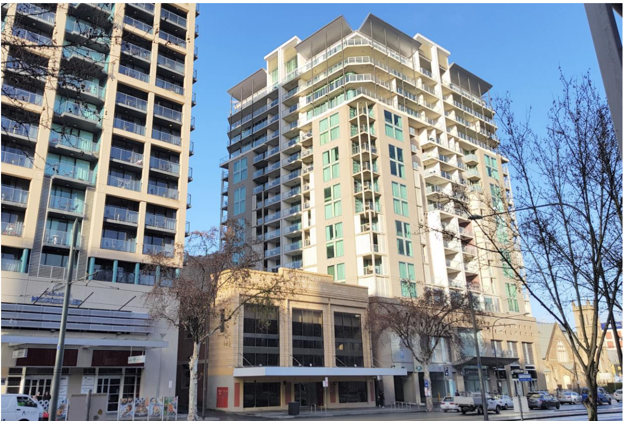
Subject land – view from northeast
