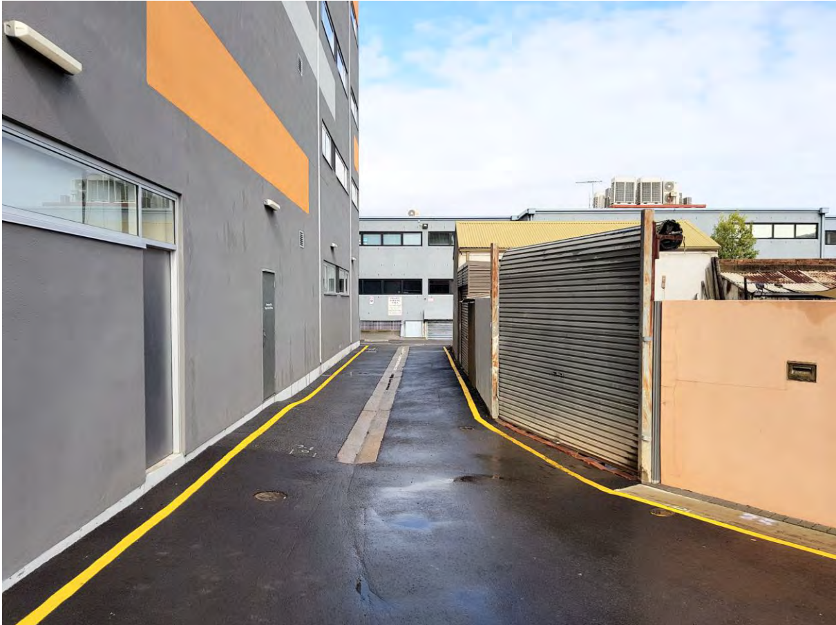
Subject Land – View to south adjacent Migrant Resource Centre (along Coglin Street west)
