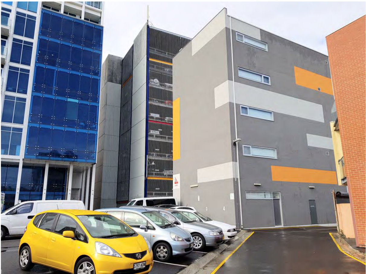
Subject Land – View to south east
