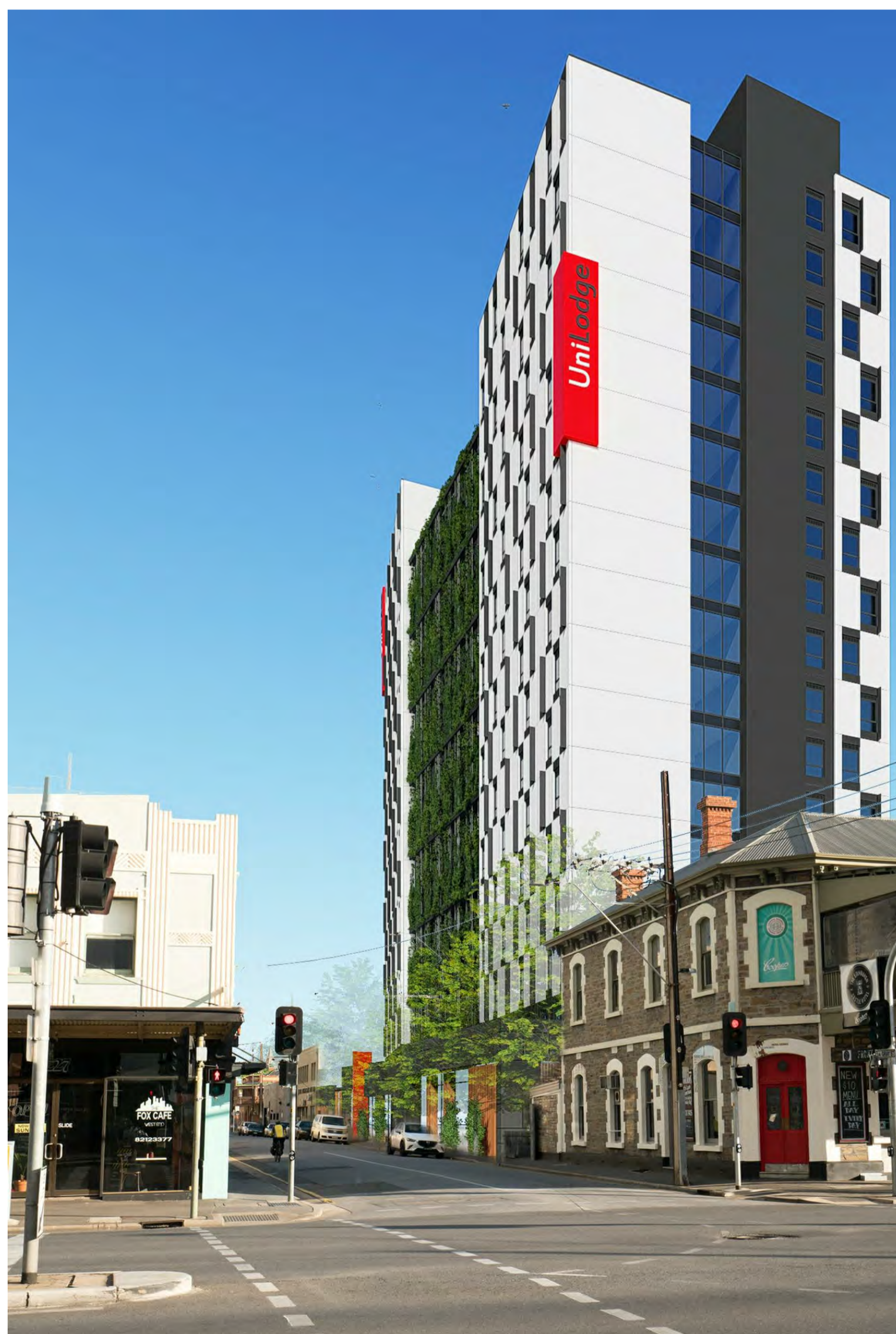
VIEW C - FROM GRAY STREET LOOKING SOUTH
