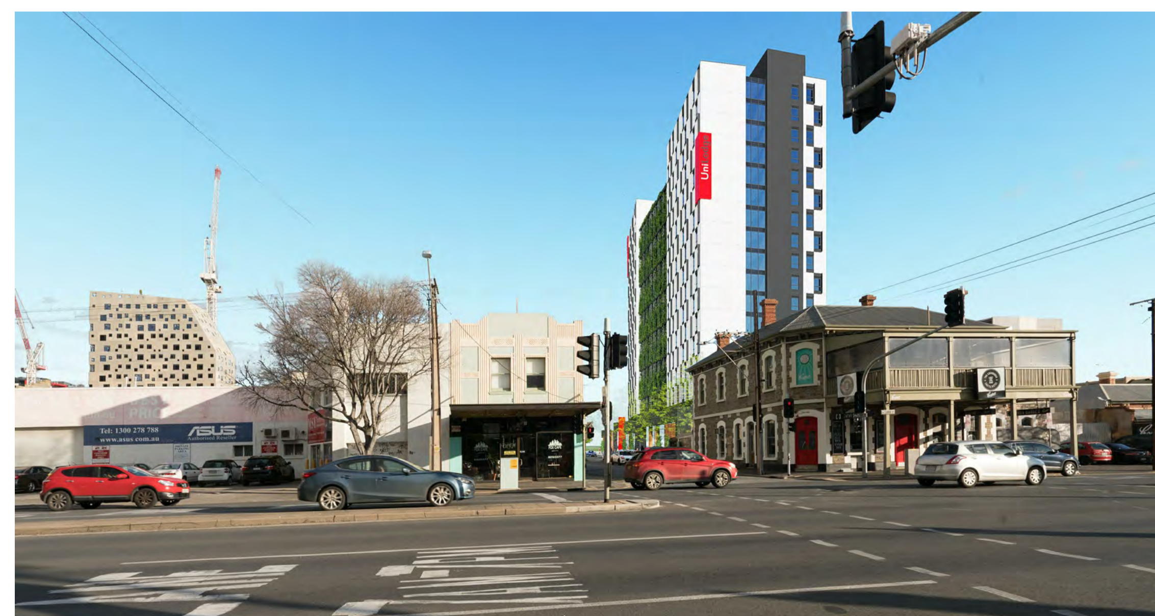
VIEW D - FROM CURRIE STREET LOOKING SOUTH
