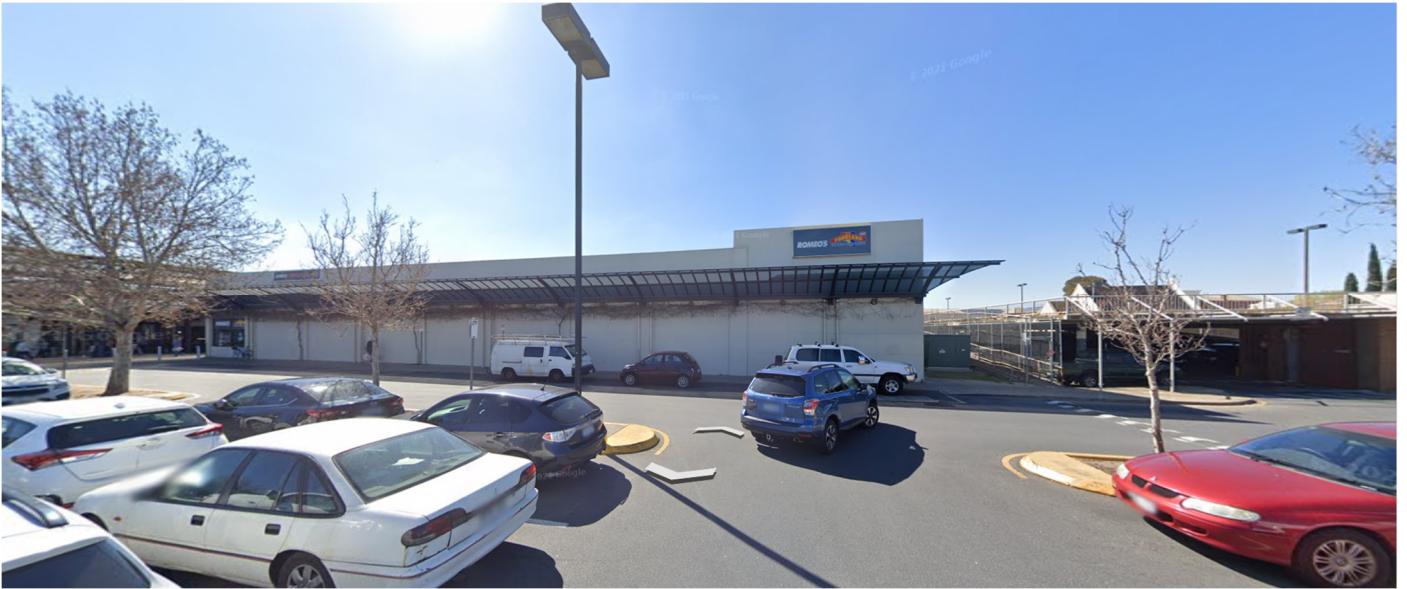
Figure 3: view from western carpark looking east, showing the eastern aspect of the existing supermarket and portion of carparking deck.
