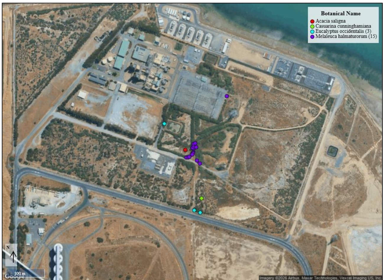
Figure 1: Pelican Point Substation
