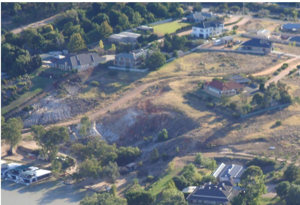
Figure 1. View of the subject land prior to the commencement of earthworks, showing the original River Murray cliff landform and natural slope before excavation.
