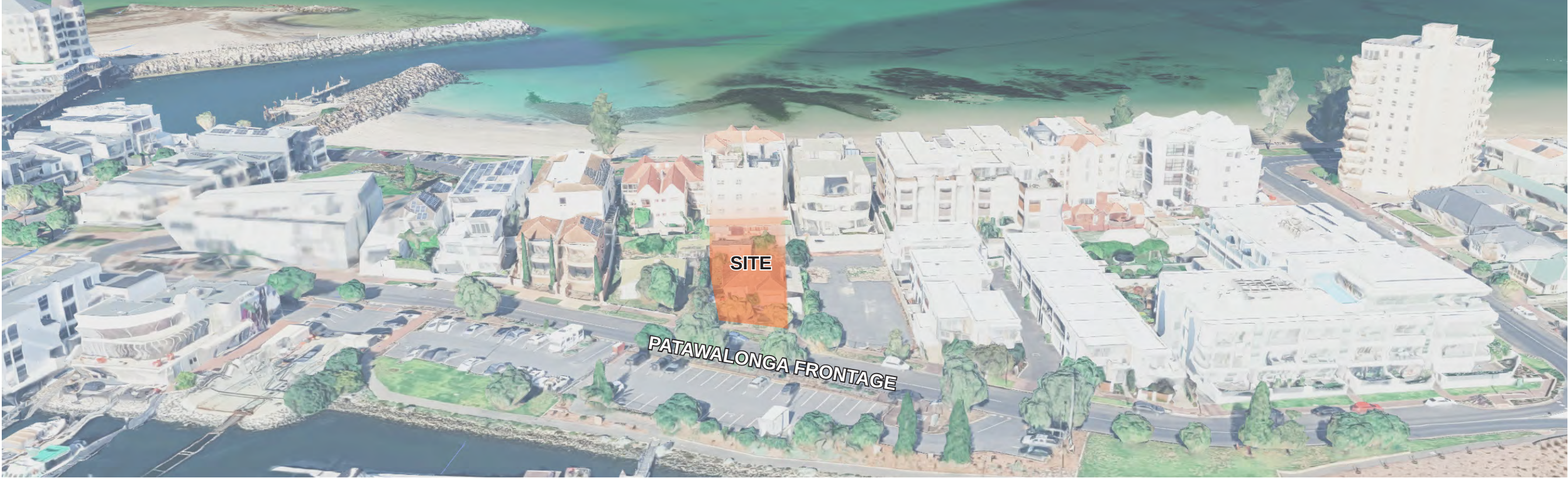
EAST AERIAL VIEW - PATAWALONGA FRONTAGE
