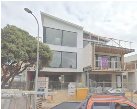
4 PATAWALONGA (UNDER CONSTRUCTION)
