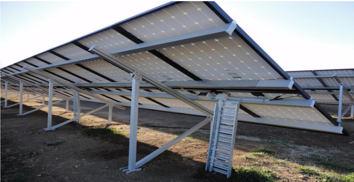
Figure 8. Typical Ground-mounted Solar Panel Layout
