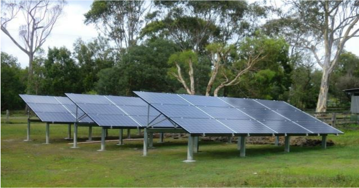
Figure 9. Typical Ground-mounted Solar Panel Layout
