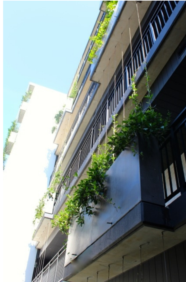
GRC planters fixed to side of East Tower Precast Walls and trained on fixed wires to detail
