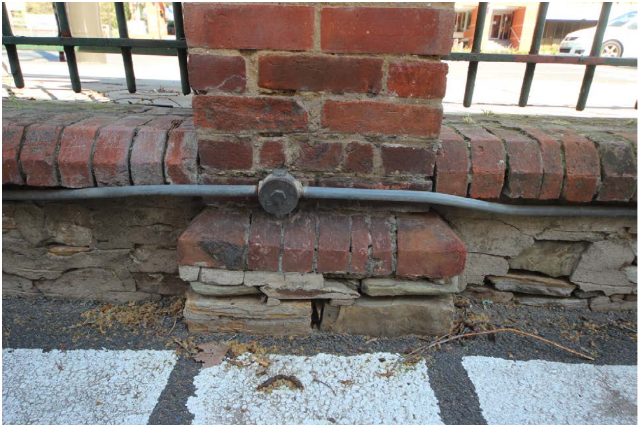
Detail view of the plinth to one of the brick pillars. Note the fretting joints in the bluestone due to the wall now acting as a retaining wall.
