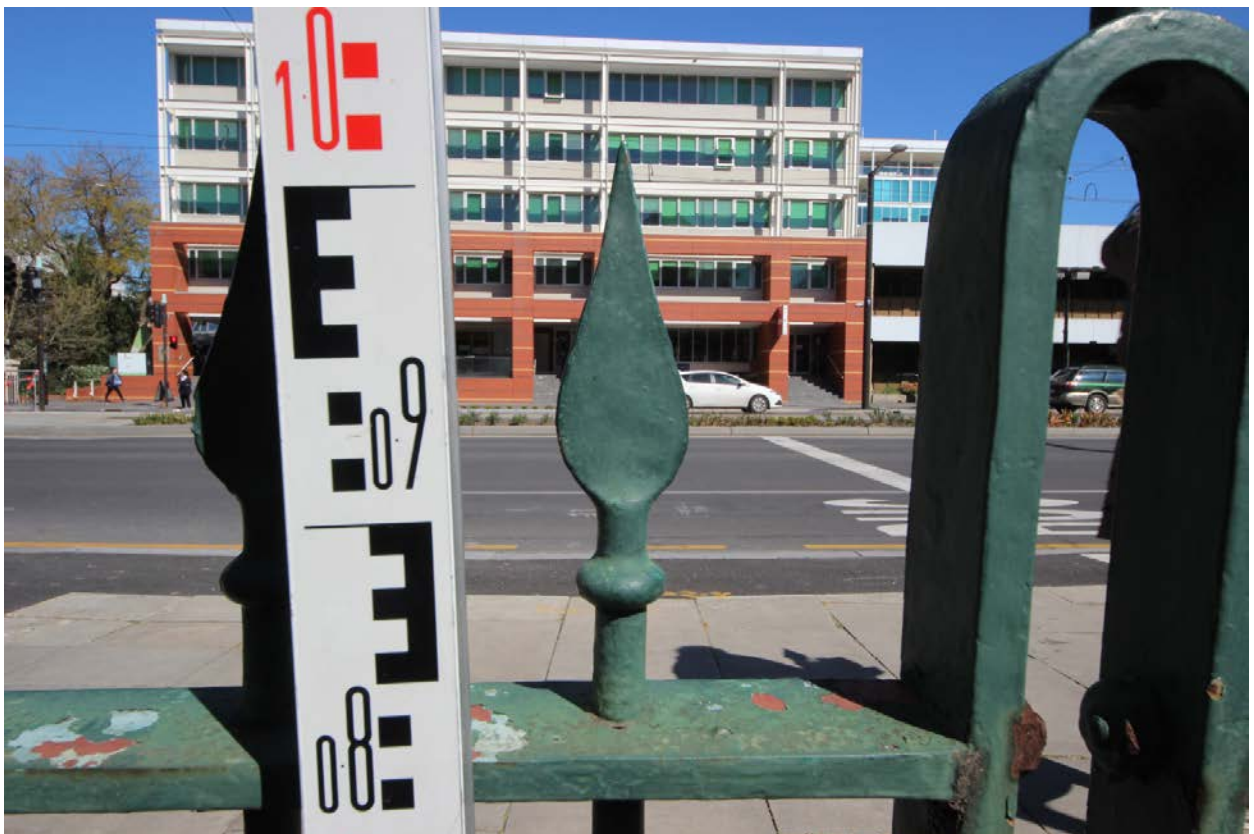
Detail of general spear top to iron railing infill.
