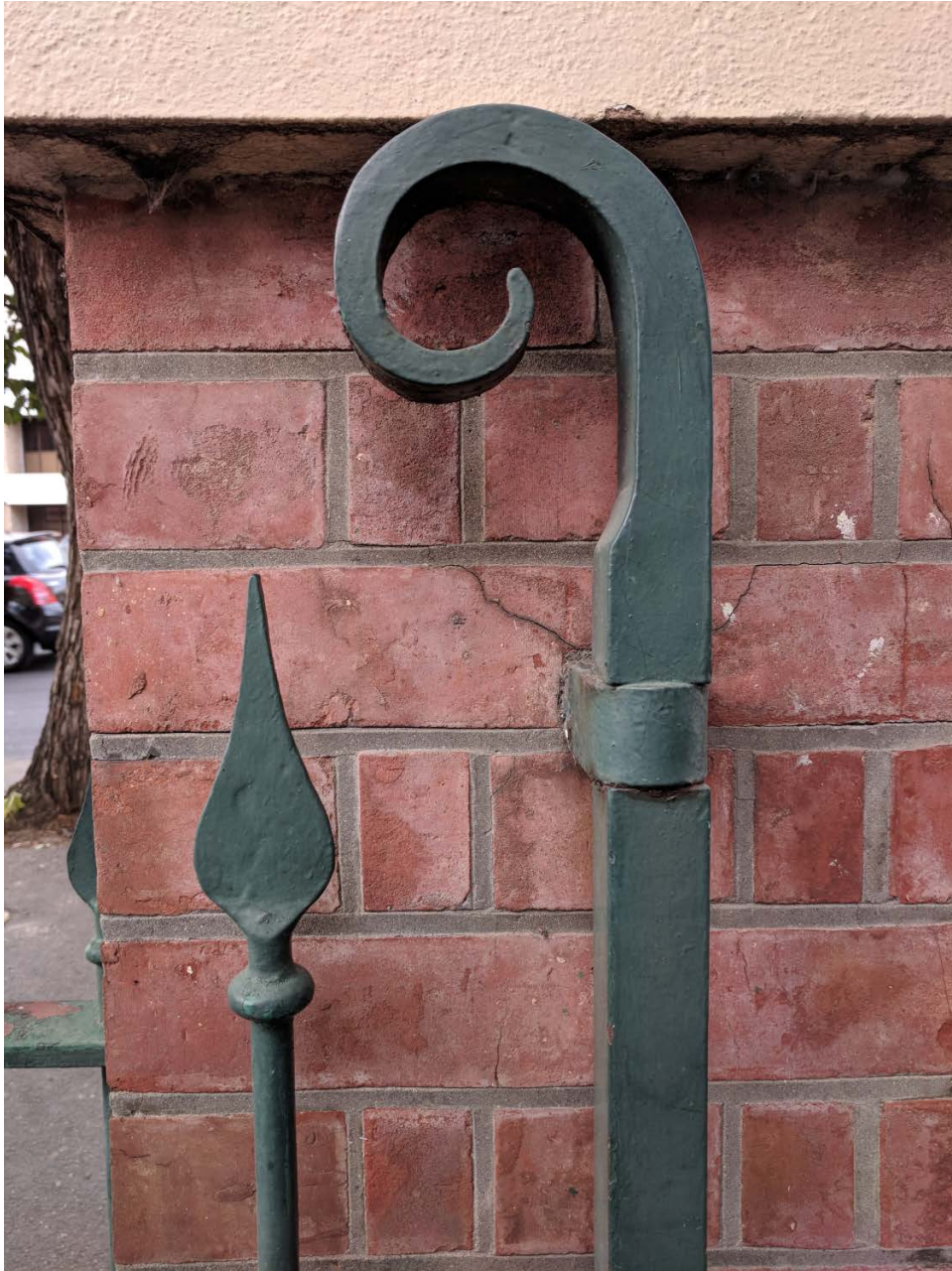
Detail view of the gate stile and a wrought spear top adjacent to the Allied Health Building.
