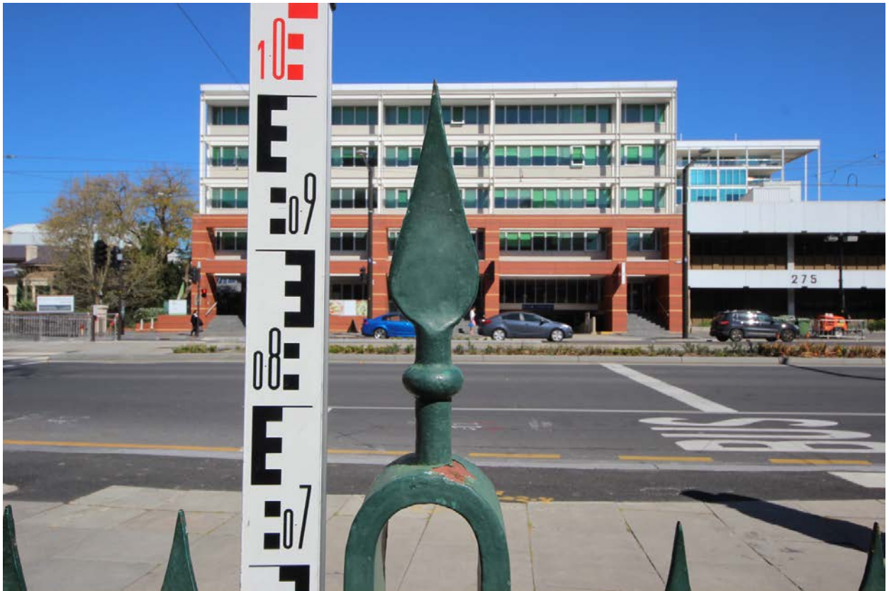
Detail view of spear on top of the hooped plate supports.
