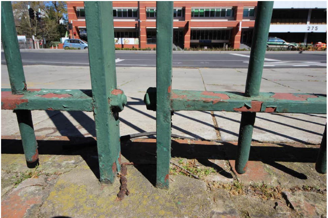
Detail view of the bolt connections of the panels to the hooped plate supports.
