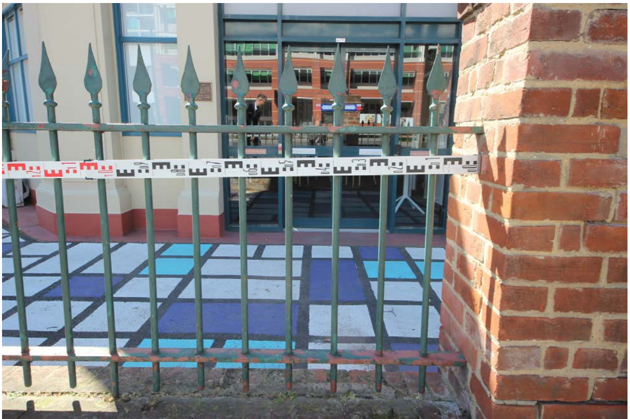
Typical wrought iron infill panel built into the brick pillars.
