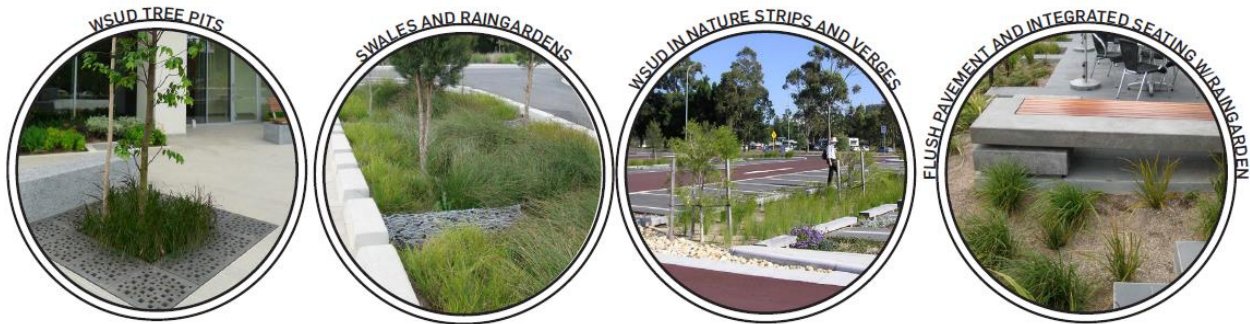
Figure 10 – Examples of proposed kerb inlet swales and raingardens
