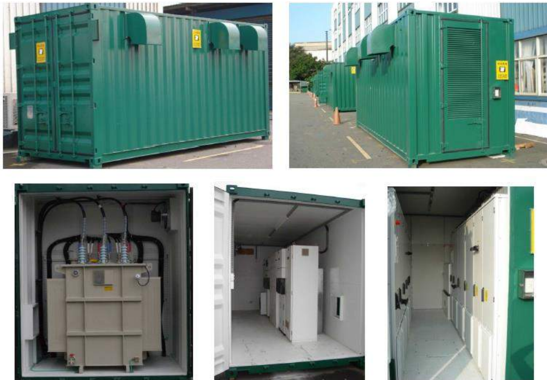
Figure 4-5 : Indicative Battery Storage Area Structure
