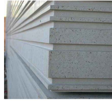
polished and textured precast concrete with horizontal recessed detailing
