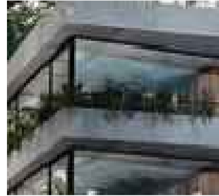
part precast & part glass balcony balustrade
