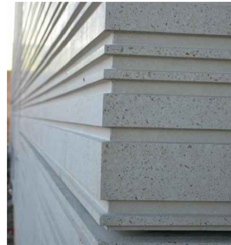
Reinterpretation - precast concrete panels with recessed detail to resemble stone and create horizontality.
