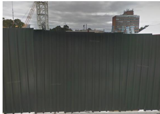
King William Street - looking north
