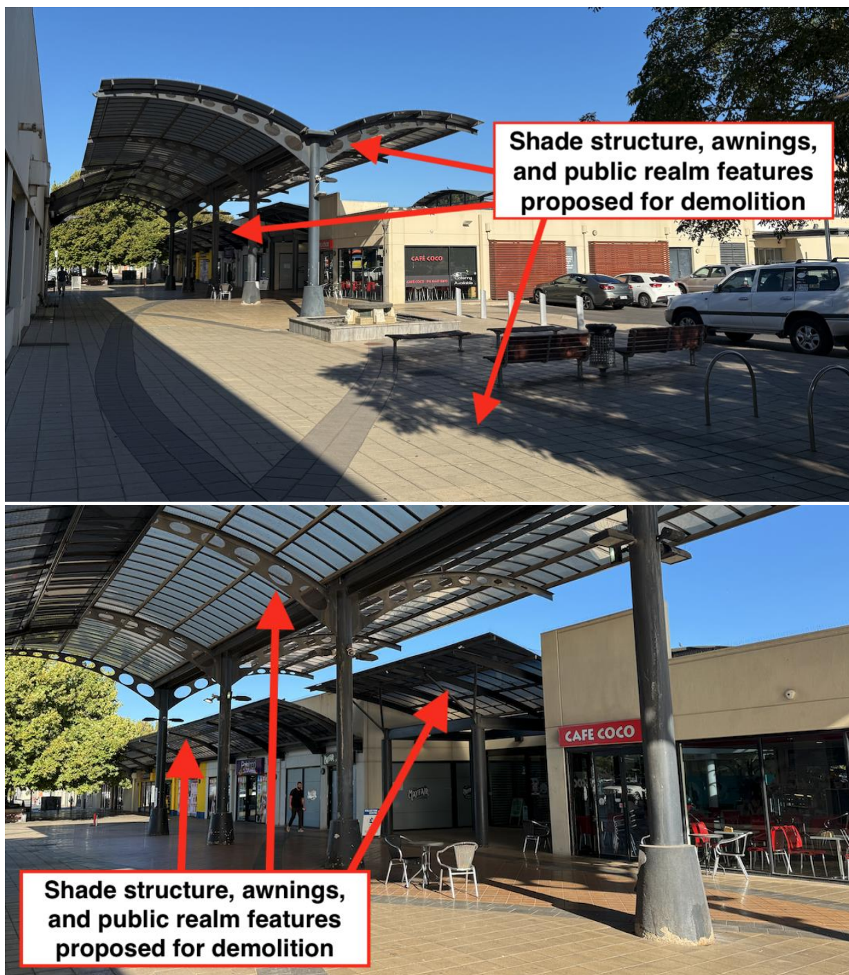
Figure 14: Public realm features on the site of the Local Heritage Place proposed for demolition.
