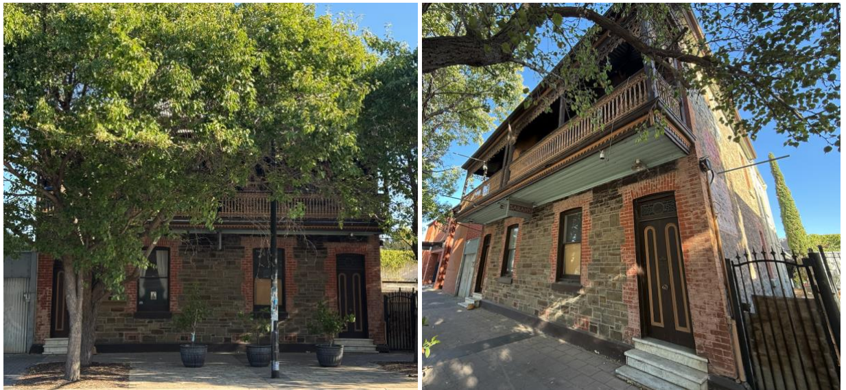
Figure 9: Semi-detached house, 85-85A Dale Street Port Adelaide (LHP) 2026
