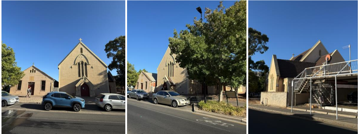
Figure 11: St Mary's Catholic Church and Hall (SHP), various views 2026
