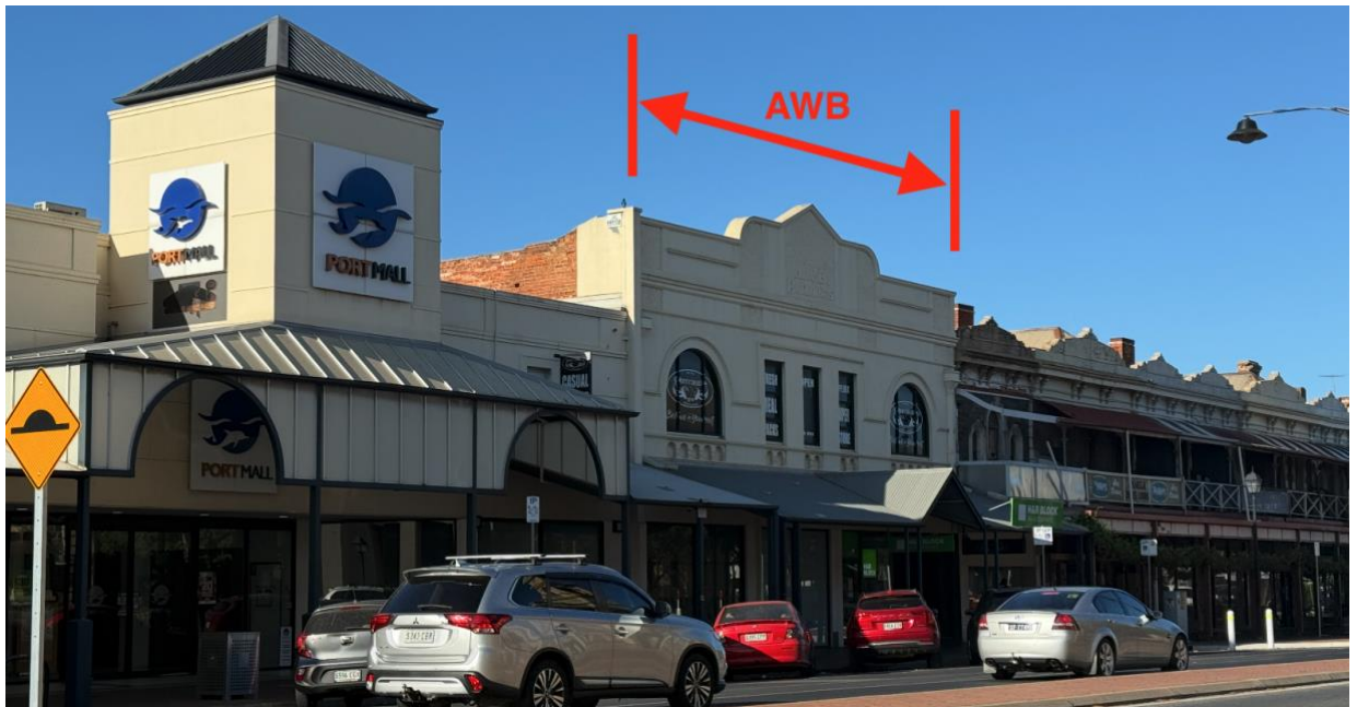
Figure 5: AWB Building set within St Vincent Street, 2026.
