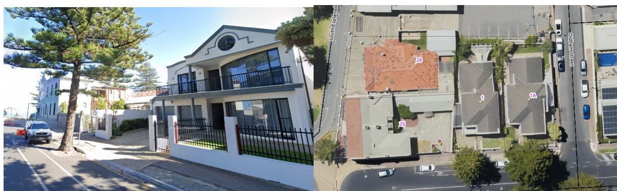
Figure 3: Pier Street Frontage (prior to demolition)
