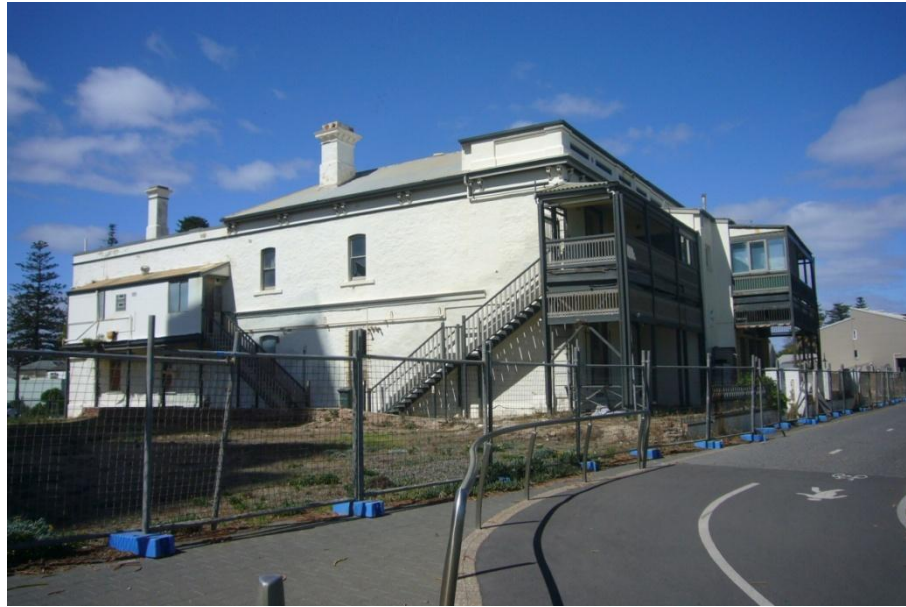
Photograph 4 : View of the much altered Local Heritage Place looking South-East
