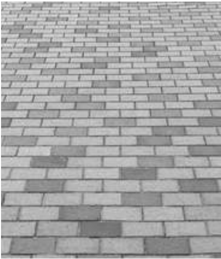
CONCRETE PAVER (3X FINISHES) TRAFFICABLE & NON-TRAFFICABLE
