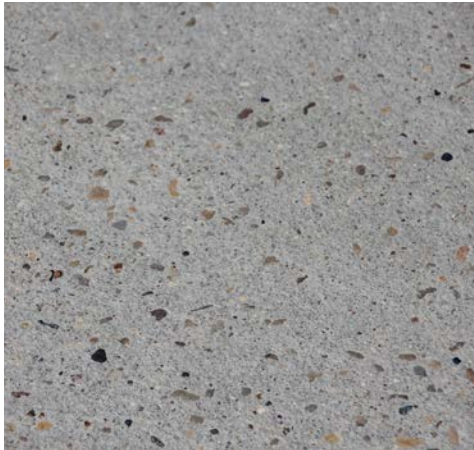
INSITU CONCRETE PAVING INSITU CONCRETE WITH LIGHTLY WASHED EXPOSED AGGREGATE FINISH USE: PATHWAYS THROUGHOUT SITE
