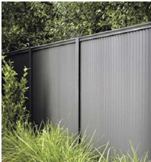
EXTERNAL BOUNDARY FENCE — 1.8m high good-neighbour fence, tapered to verge — Neutral panel colour. Articulated post colour.
