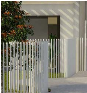
PALISADE FENCE (1200) — High quality semi-permeable boundary fence. — 1.2m high to cafe/kiosk courtyard
