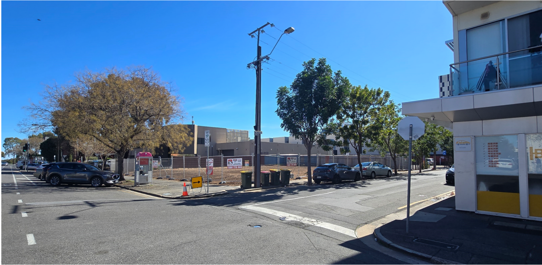
Figure 2.2 - Site Photograph taken August 2025, received from PACT Architects.
