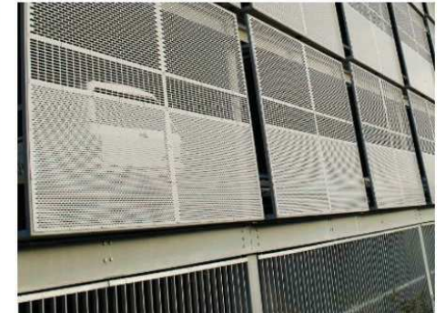
04 - PERFORATED ALUMINIUM SCREEN ON FULLY WELDED SHS FRAME TO MATCH EXISTING
