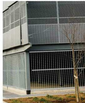
06 - HOT DIPPED GALVANISED BAR SCREEN ON FULLY WELDED STEEL FRAME
