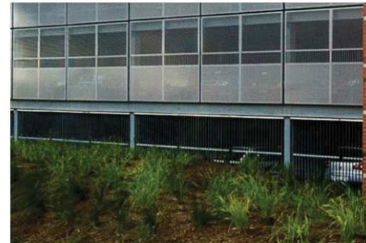
05 - ZINCALUME FINISH MINI-ORB CORRUGATED METAL SHEET SOFFIT
