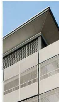
05 - ZINCALUME FINISH MINI-ORB CORRUGATED METAL SHEET SOFFIT
