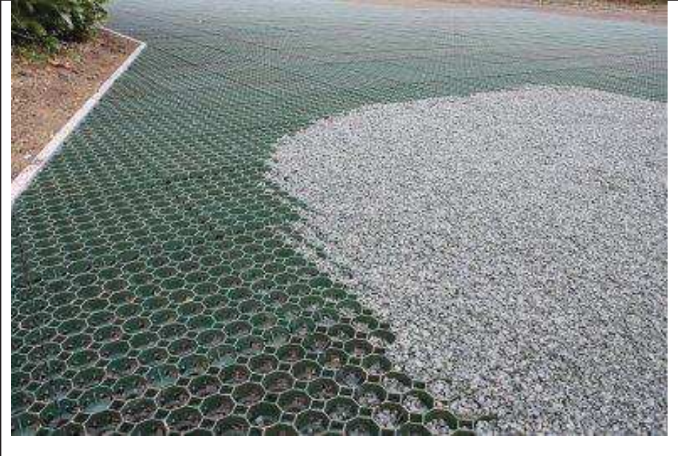
Use of Eco cell structure over the driveway using 20mm gravel (Non-Fines) between cells.
