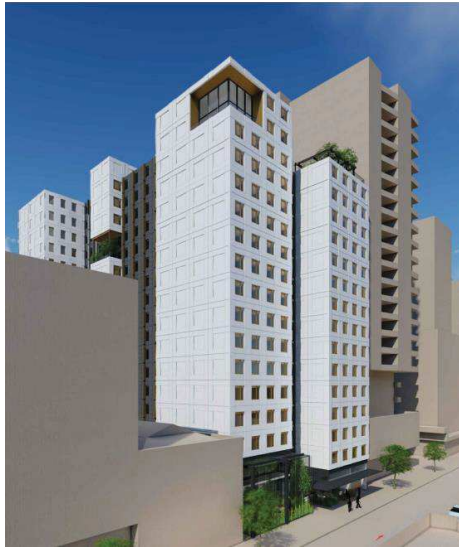
Figure 6: The low glazing-to-façade area ratio results in a high thermal mass content, which helps to stabilise internal temperatures.
