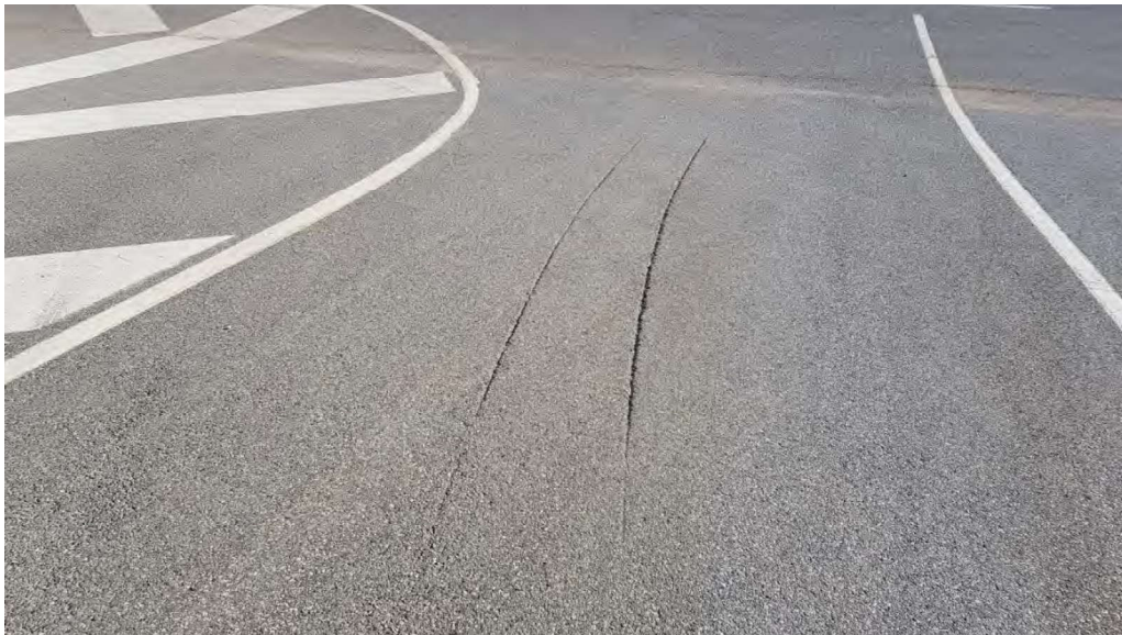
Figure 4-9 - Gauge marks at the access point
