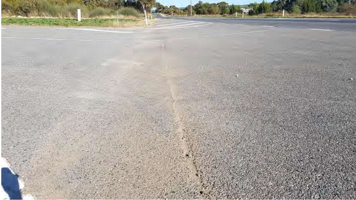
Figure 4-11 - Erosion across the face of the access point
