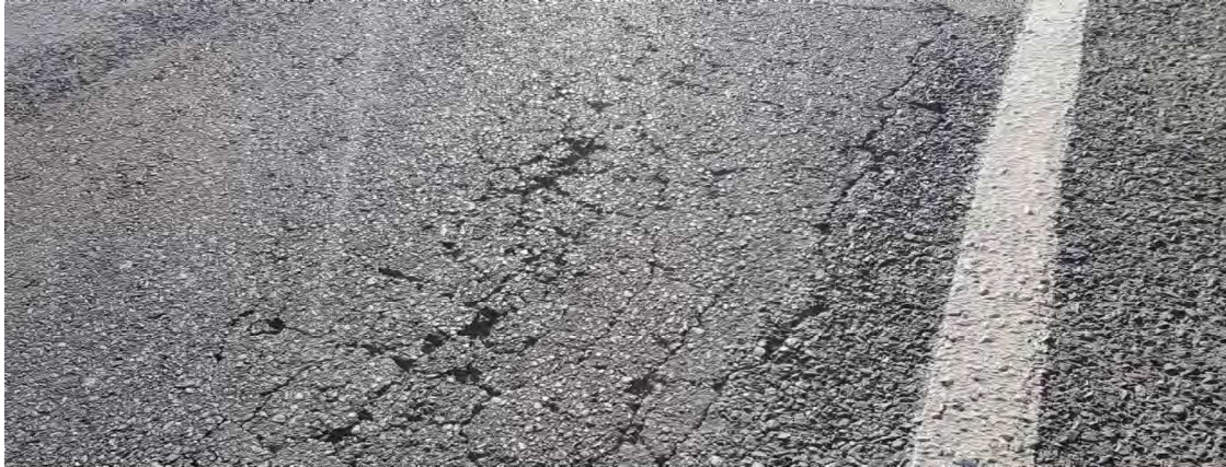
Figure 4-6 - Crocodile cracking on Callington Road
