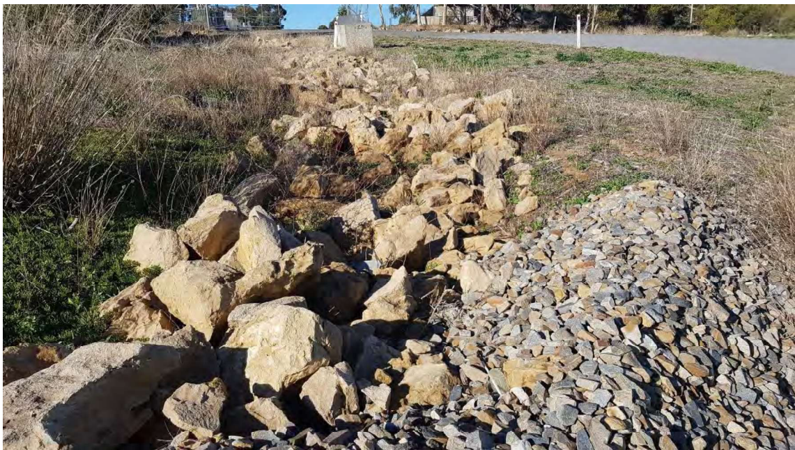
Figure 4-12 - Rock-lined swales alongside the access point
