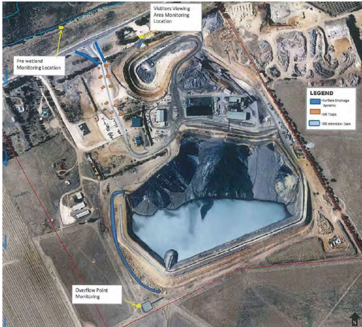
Figure 15: Stormwater management (source: Terramin, 2017)
