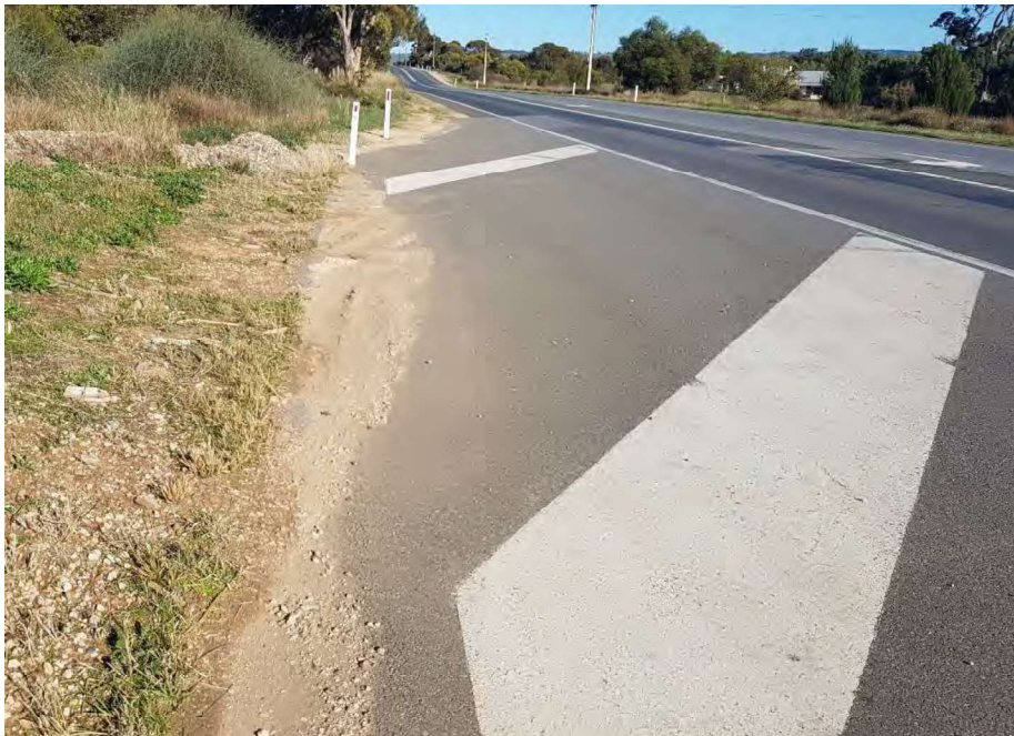
Figure 4-10 - Silt and minor deformation along Callington Road
