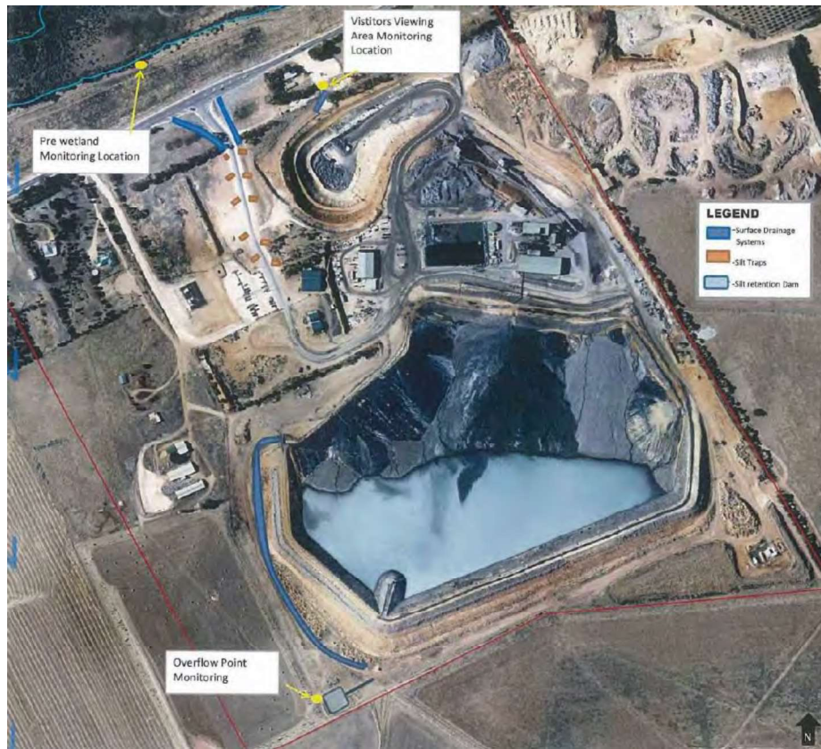
Figure 3: Surface water drainage infrastructure
