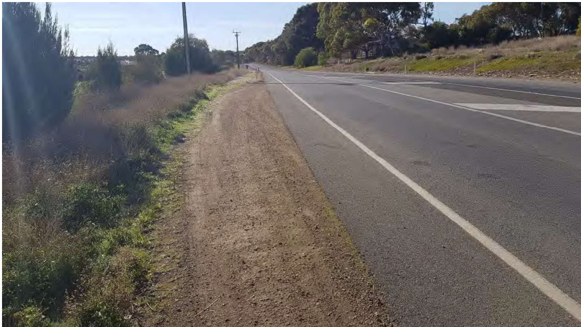
Figure 4-7 - Vehicle track marks off the sealed shoulder of Callington Road
