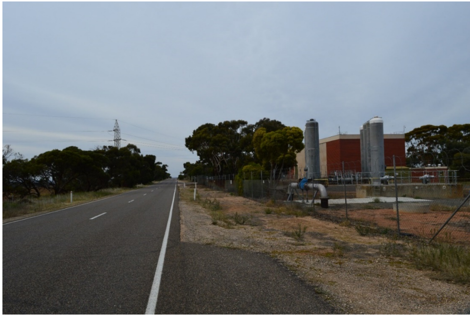
View of the SA Water pumping station on the southern side of Monarto Road, opposite the subject land.
