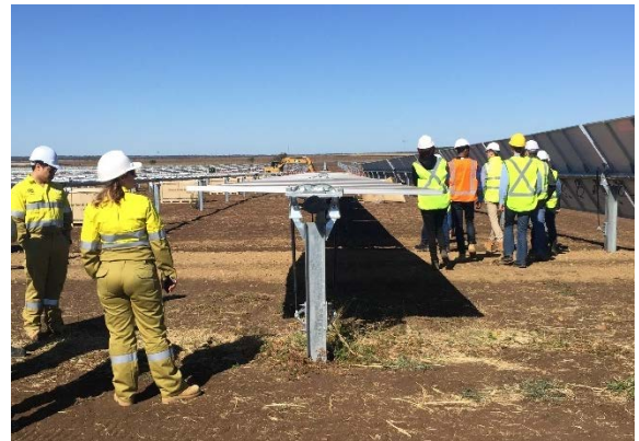
Photographs of construction and installation of single axis photovoltaic panels at RES' Emerald Solar Farm in Queensland.
