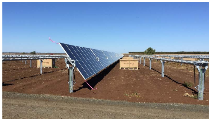
Photographs of construction and installation of single axis photovoltaic panels at RES' Emerald Solar Farm in Queensland.
