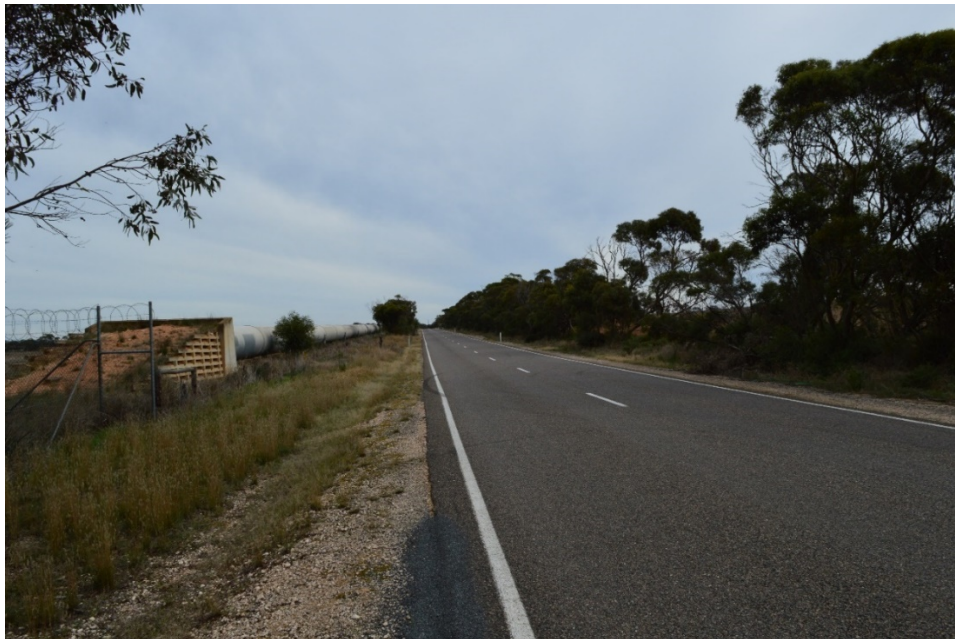
View of SA Water pipeline adjacent Monarto Road and opposite the subject land.
