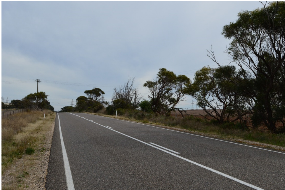
Photograph taken from Monarto Road, looking in a westerly direction, with the subject land to the right of the photograph. Some of the 33kV and 132kV infrastructure on the subject land is evident in the photograph, as is existing roadside vegetation.
