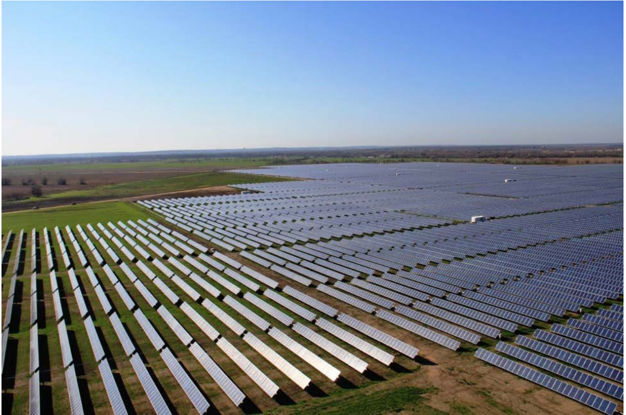
Photograph of a typical array of single axis tracker photovoltaic panels in a solar farm.
