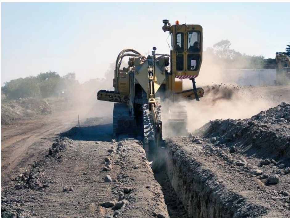
Plate 6.14: Underground Reticulation Cable Trenching Machine
