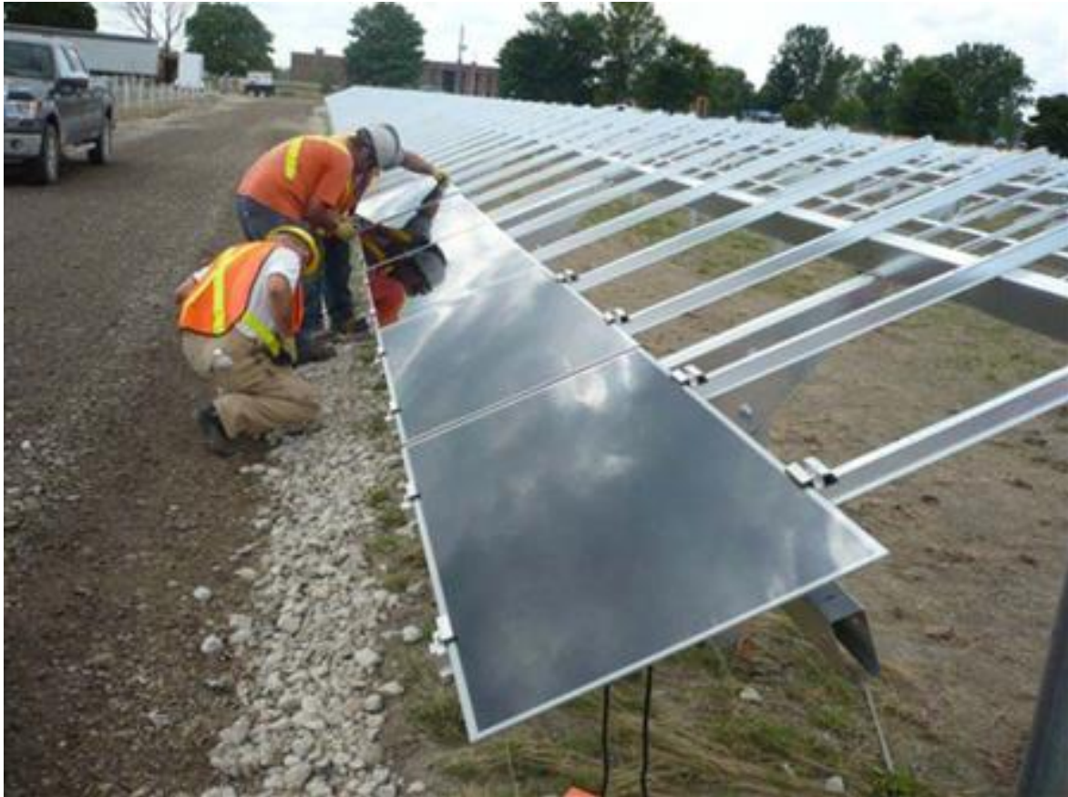
Plate 6.10: Installing Modules on Framework
