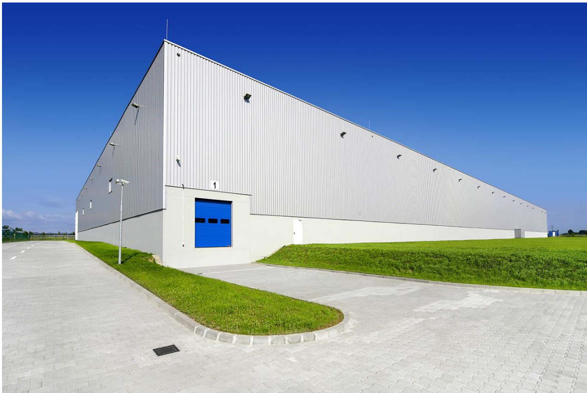
Plate 6.4: Example Energy Storage Building
