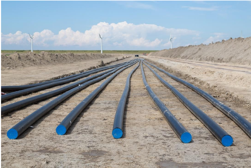
Plate 6.7: Typical Underground Cable Arrangement
