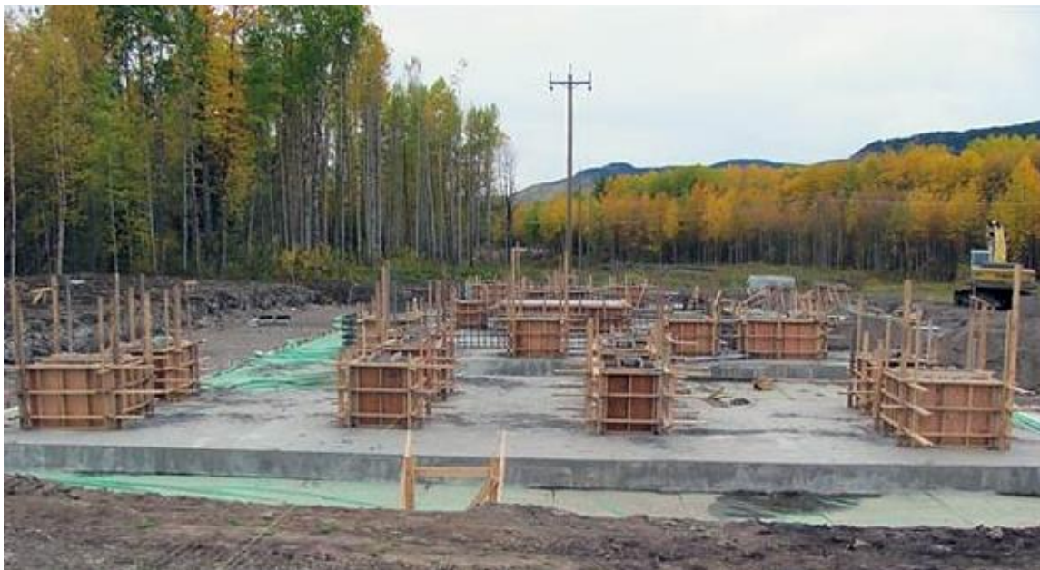
Plate 6.11: Typical Substation Foundations
