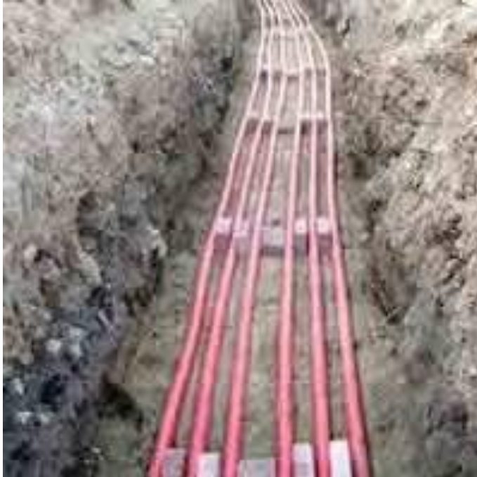
Plate 6.13: Example Export Cable Trench
