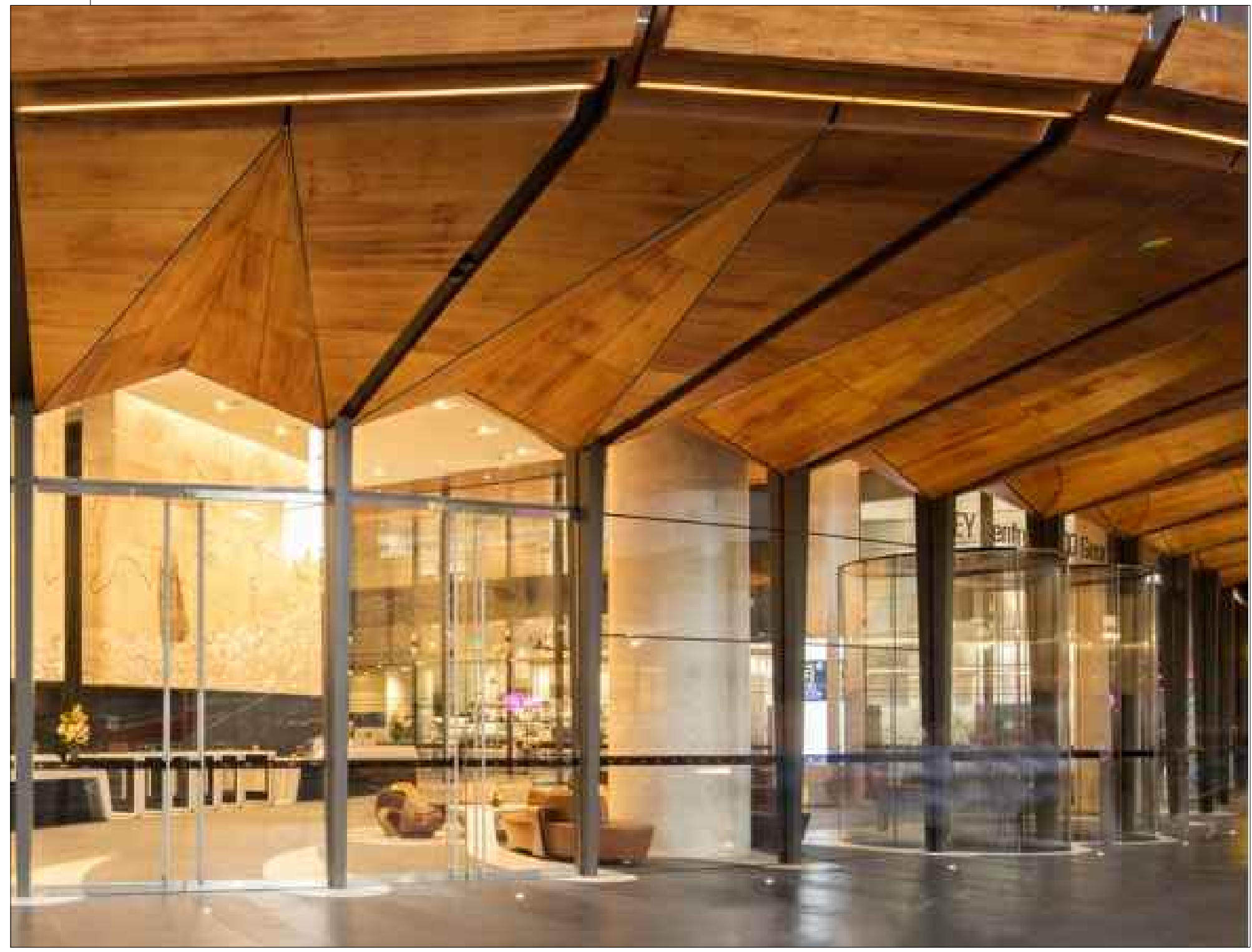
marine ply soffit
