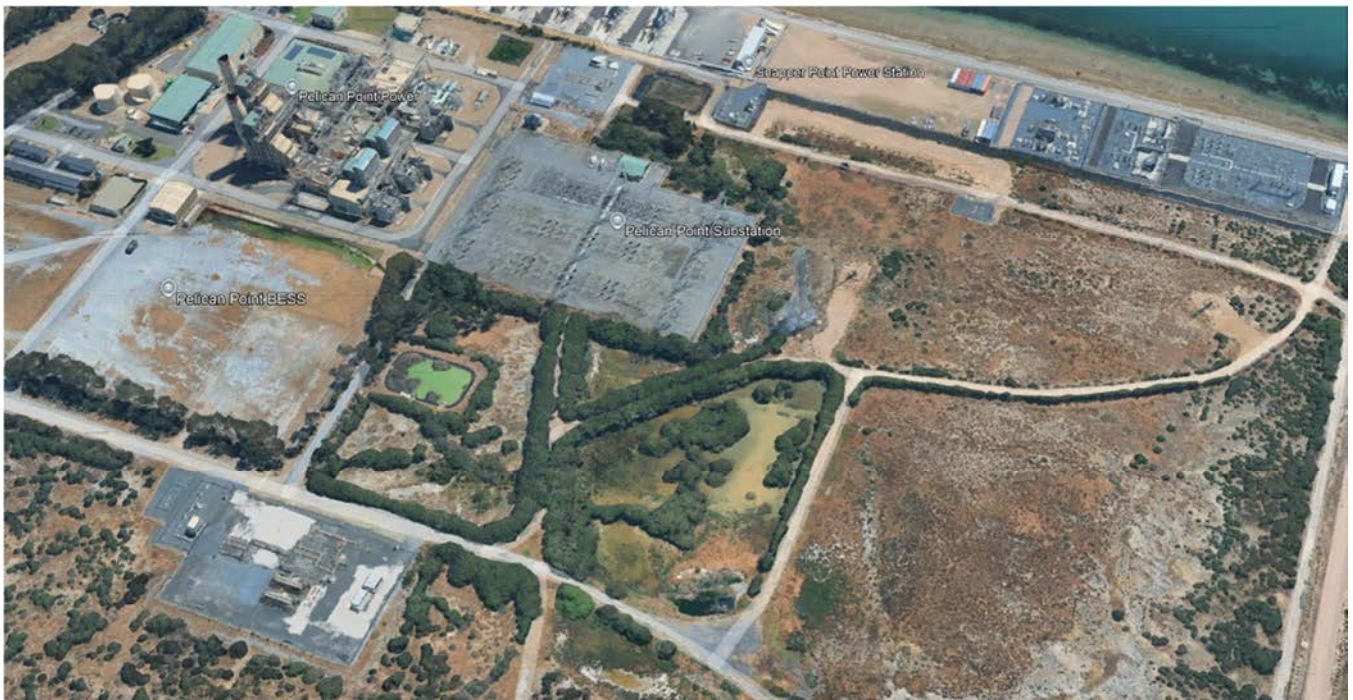
Figure 12: Aerial Photo Pelican Point Substation Site looking north toward Port River (Source: Google Earth)
