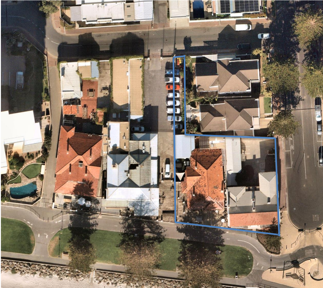
Photo 5: Aerial view of the previous site prior to demolition of the former short stay accommodation buildings.
