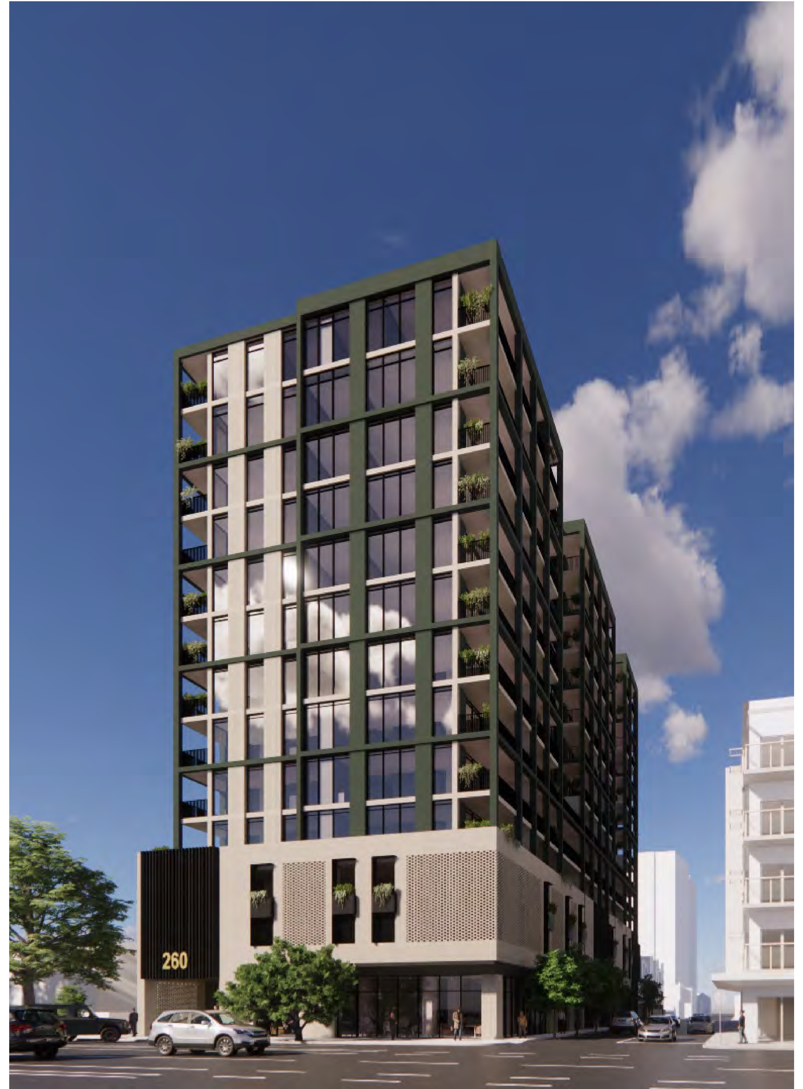
View of South Facade from Franklin Street
