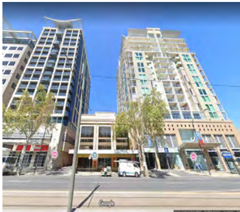
North Terrace - looking south toward subject site Figure 3 - Site Photos, sourced from Google Maps
