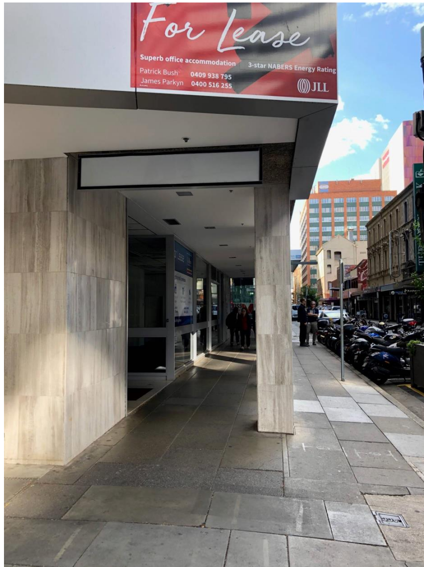
View of existing setback of 50 Pirie Street to Gawler Place (building to north of subject site)
