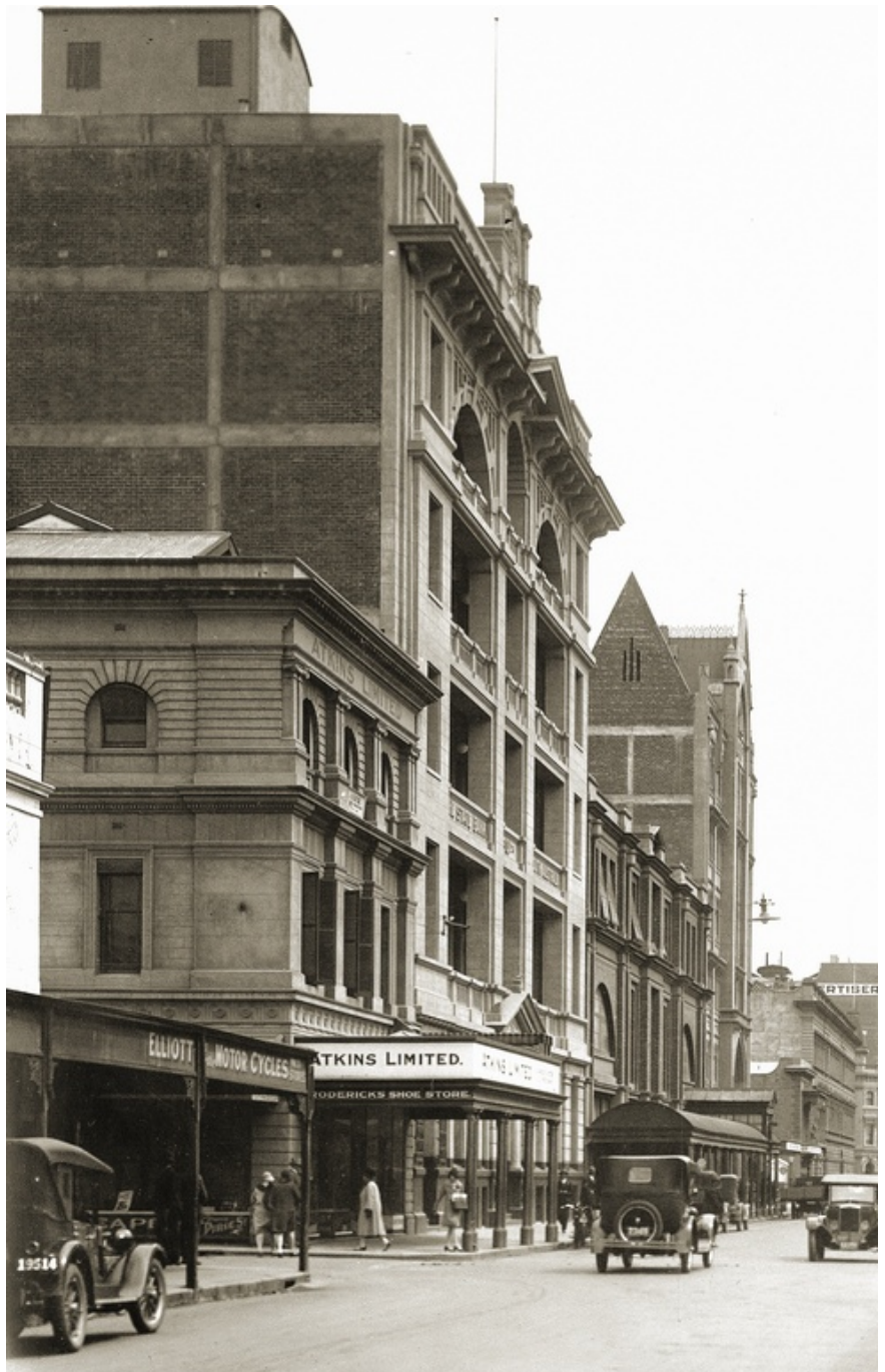
Figure 4: Former State Bank of South Australia, c1928. Source: SLSA, B_5187
