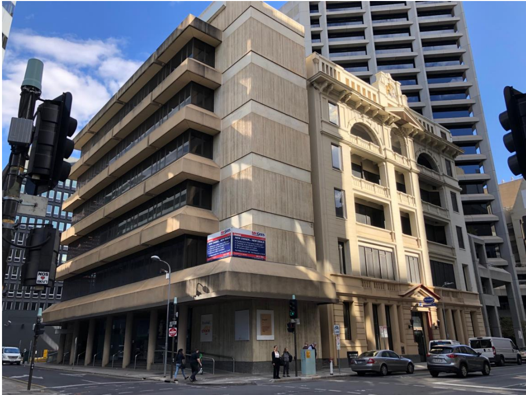
51 Pirie Street – from diagonally opposite corner
