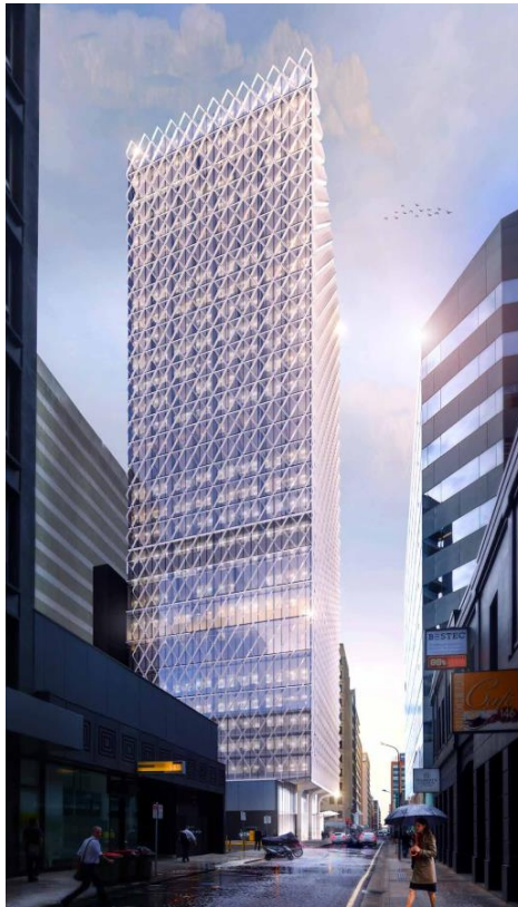
Figure 6: Highly glazed façade maximises daylight to guest rooms and areas (Image courtesy of GHD WOODHEAD)
