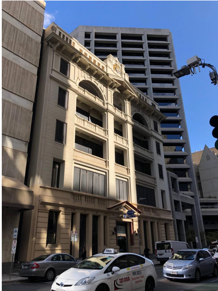
View of Local Heritage (Townscape) Place Photograph shows modern alterations to façade
