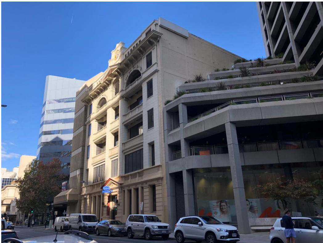
View of 51 Pirie Street from northern side of Pirie Street
