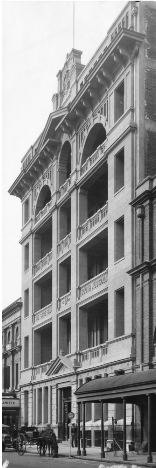
Figure 5: Former State Bank of South Australia, c1928. Source: SLSA, B_4716
