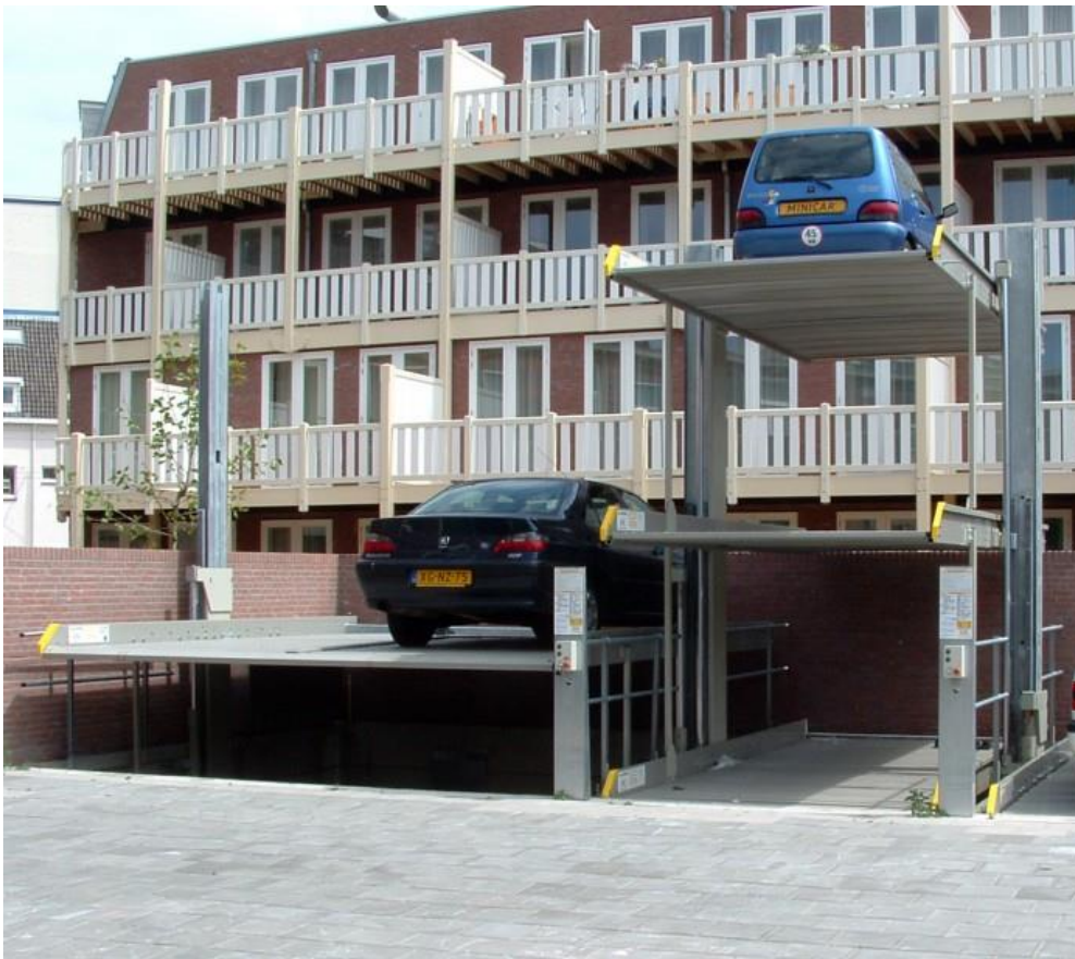
Figure 2: Parklift 413 three-level stacker system (Source: Wohr website)
