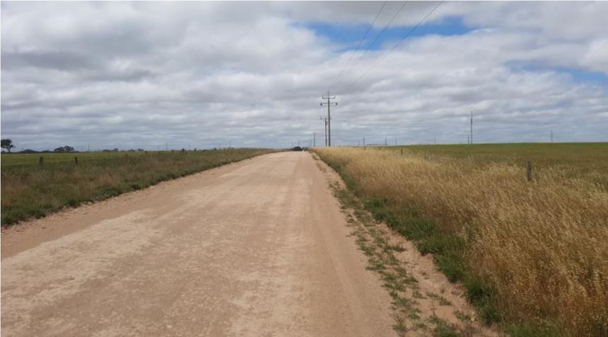
Plate 4-4 Substation Road, located adjacent to subject site
