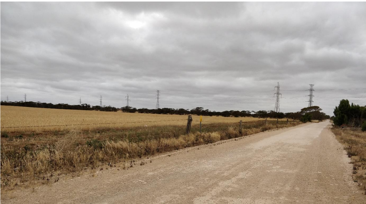
Plate 4-3 View of subject site from Substation Road, showing high voltage transmission lines and patches of vegetation
