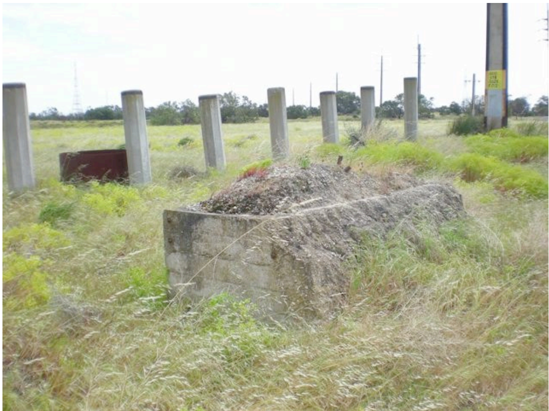
Figure 13 Detail of eastern feature at Site 1 to north. DSCN 2599
