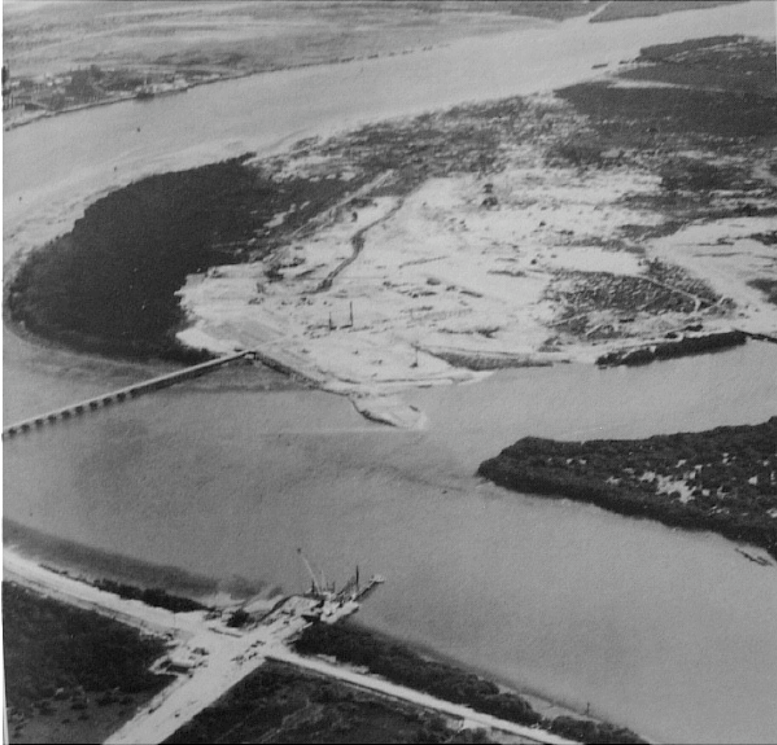
Figure 9 Aerial view of the power station site, c. 1963. (Source: Linn 1996, p. 139)
