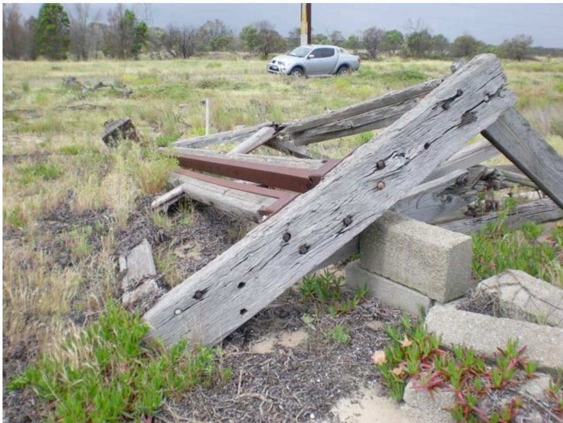
Figure 17 Detail view of the pile driver at Site 2 to the southeast. Note the steel guides fixed to the main timbers and the besser-style blocks. DSCN 2625
