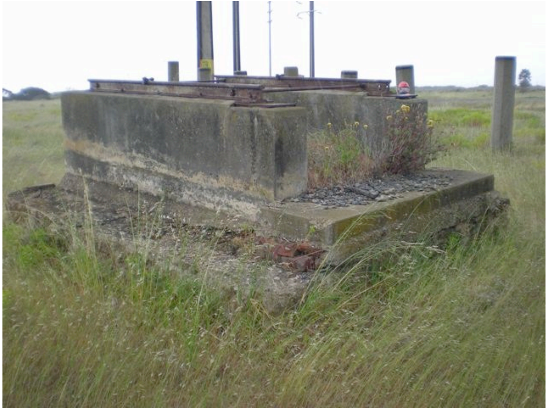
Figure 14 Detail of western feature at Site 1 to northeast. DSCN 2605
