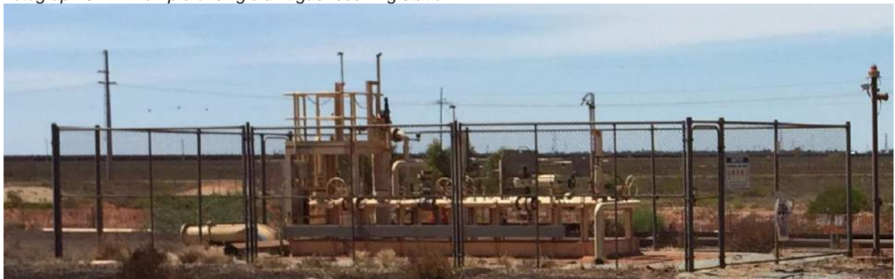
Photograph 6-1 - Example of single unit gas receiving station
