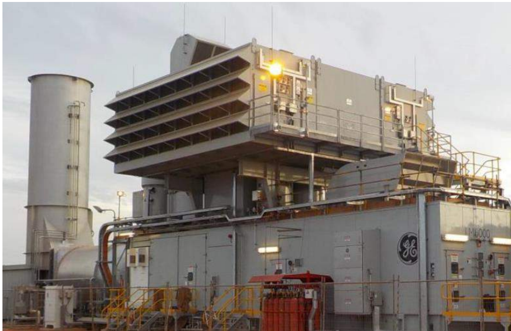
Figure 6-7 - LM6000 generator package at Alinta Energy's Boodarie Power station during construction
