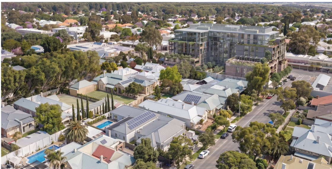
Figure 2 View of site and locality from eastern aspect
