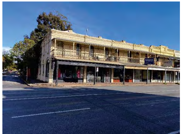
Photograph 5 View looking offsite to the west towards the former dry cleaning location
