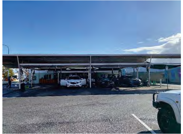
Photograph 4 View looking offsite to the north of the car wash business
