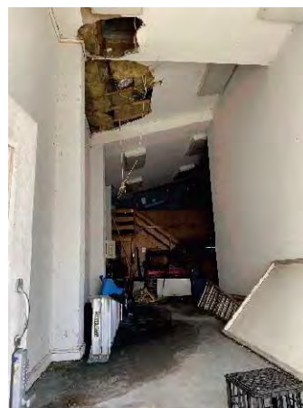
Photograph 6 View taken from the northeast corner looking inside the large building along the eastern boundary
