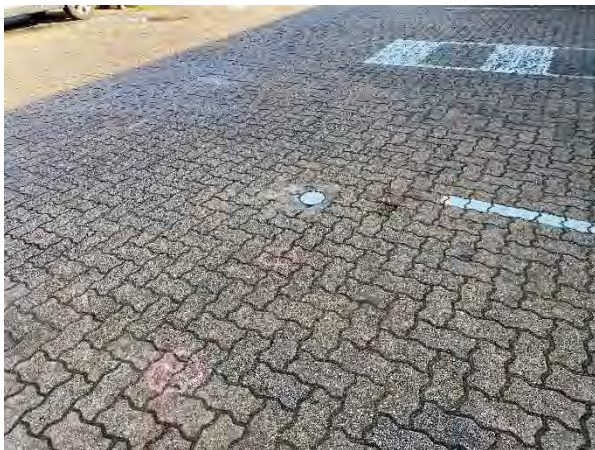
Photograph 2 View of the groundwater monitoring well on the southeast portion
